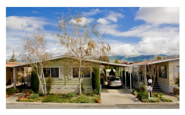
HUD "Manufactured Home Construction and Safety Standards (3280)". It may be installed on a temporary or permanent foundation. A transportable home built on a permanent chassis prior to June 15, 1976, is a "mobile home" and the acceptance of the design and construction of a mobile home is up to the local jurisdiction.
