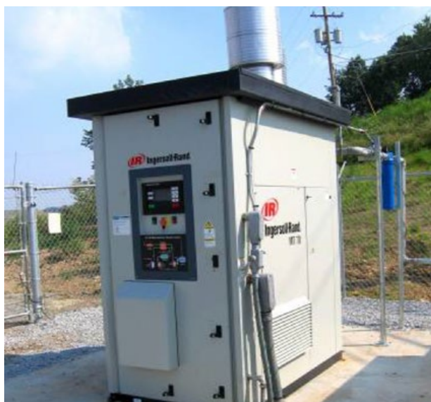
FIGURE 1-10: BAILEY MINE MICROTURBINE (SOURCE: INGERSOLL RAND)
