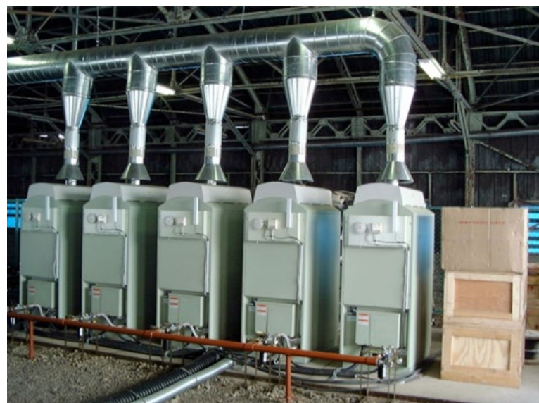
FIGURE 1-11: MICROTURBINES OPERATING AT ABANDONED AKABIRA MINE IN JAPAN (SOURCE: U.S. EPA)
