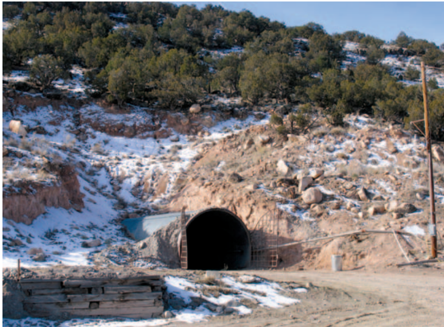
Figure 38. Portal of the West Sunday Mine, in the Sunday-Saint Jude Mine Complex of Denison Mines, Inc., San Miguel County. (Photo by Chris Carroll).
