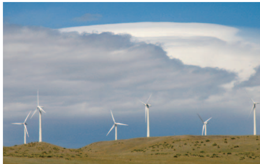
Figure 40. Ponnequin Wind Farm, Weld County.
