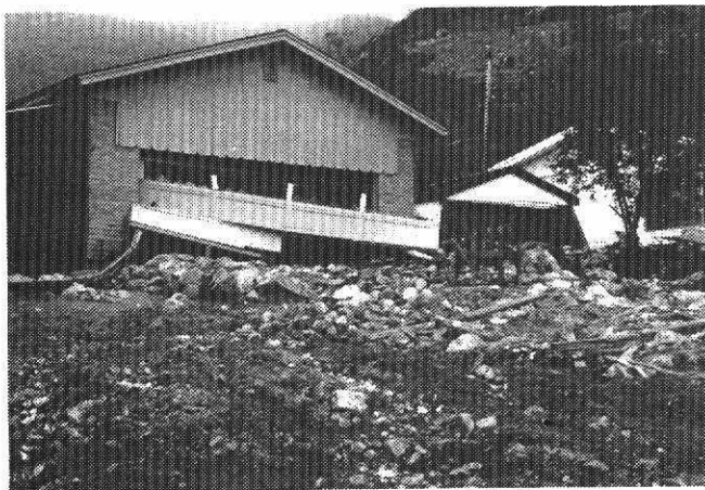
Figure 2. Major damage to homes in Farmington, Utah as a result of 1983 Rudd Creek mudslide (photograph by Robert Kistner, Kistner and Associates).
