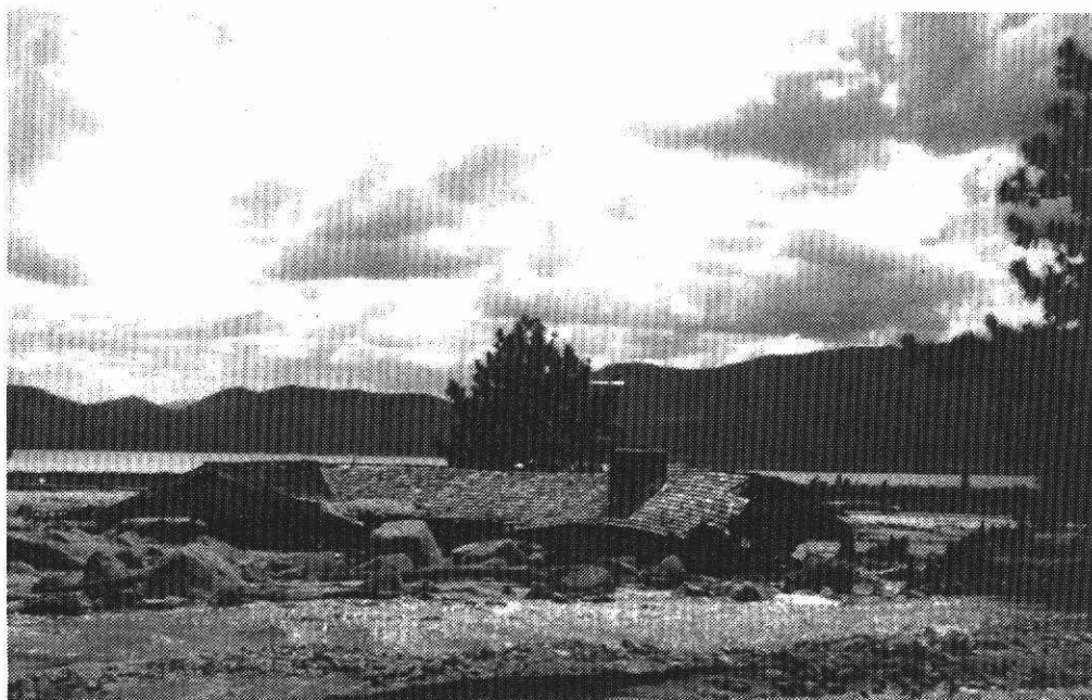
Figure 17. House destroyed by 1983 Slide Mountain, Nevada landslide (photograph by Robert J. Watters, University of Nevada, Reno).
