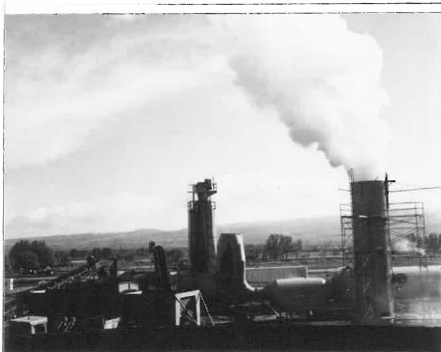
Photograph No. 10 First day of production. Note scaffolding set up next to stack for stack particulate monitoring.
