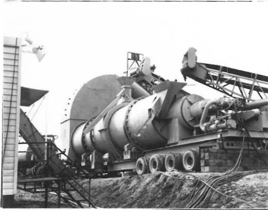
Photograph No. 9 View of CMI 9' X 36' Recycle Plant used on Project.
