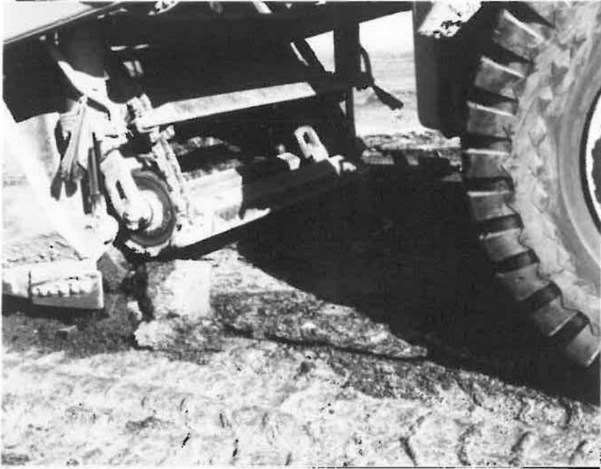
Photograph No. 1 Scraper picking up old pavement from roadway
