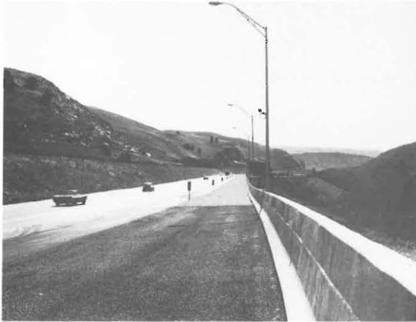
Looking down the escape ramp from the paved approach toward the gravel arrester bed. NOTE POLE MOUNTED VIDEO CAMERA.
