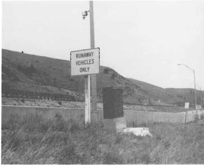
View from behind the retaining wall showing the location of the video equipment cabinet.
