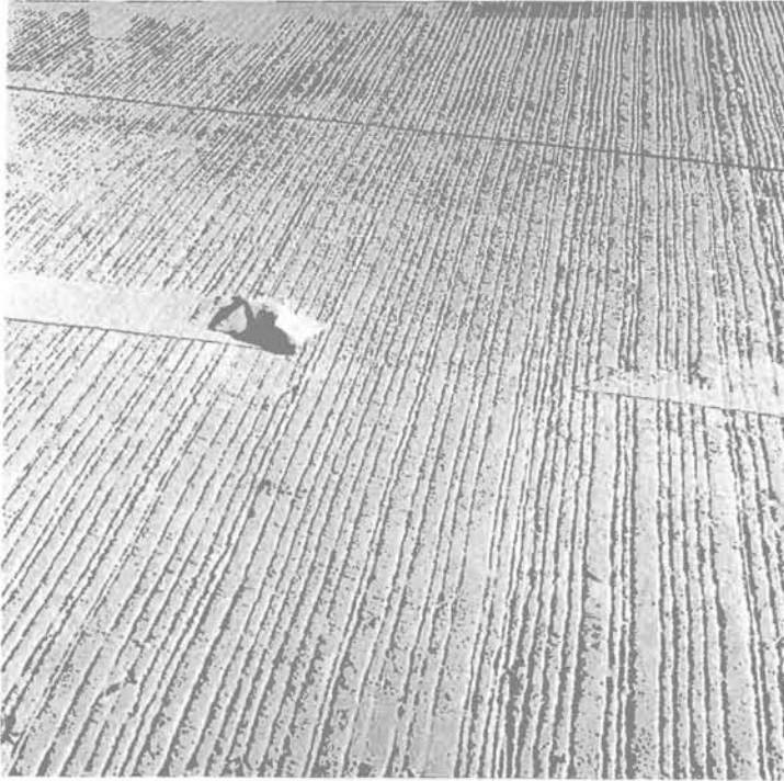
Area where snow plow blade has peeled back the plastic pavement marking.
