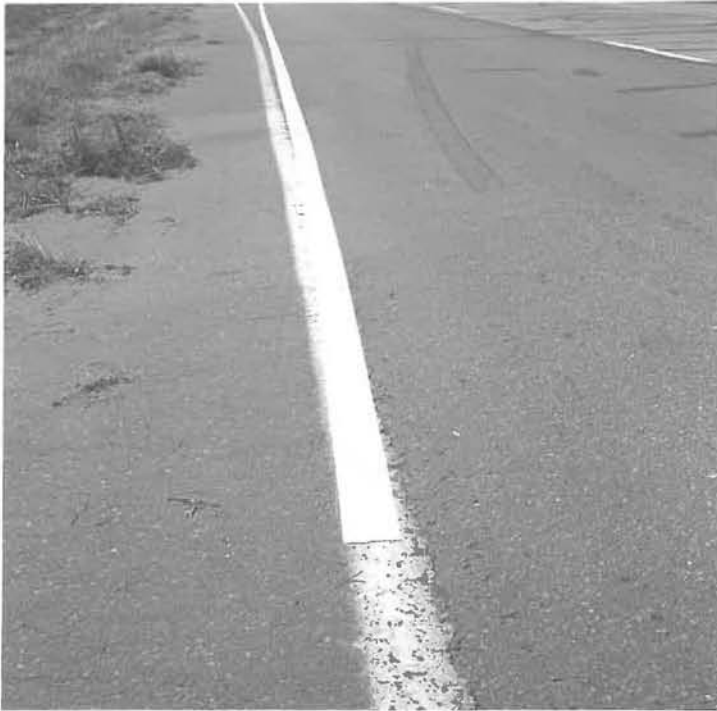
Striping applied at beginning of turnout.
