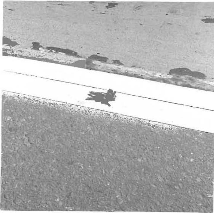
Double width striping applied where required.
