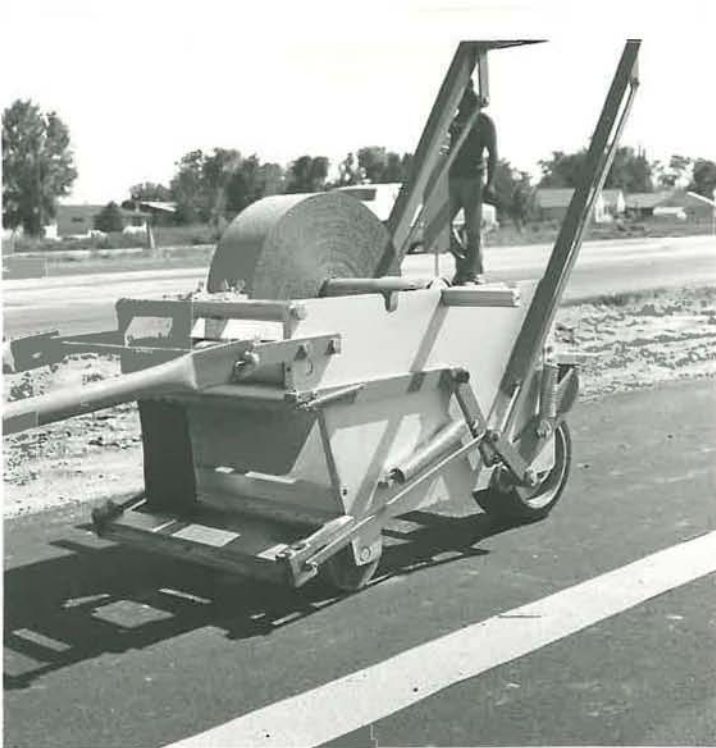
Close up view of Marking tape applicator
