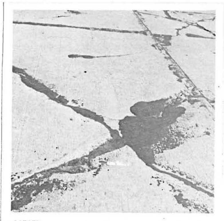
Area where centerline striping has been removed. No residue remains.
