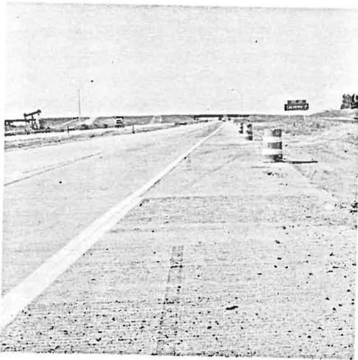
Area showing where center-line striping has been removed from concrete pavement.
