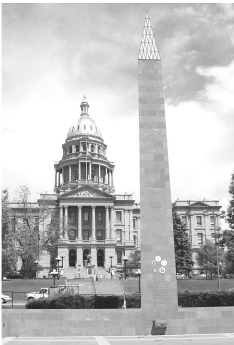
Colorado State Capitol is constructed with Aberdeen Granite from Gunnison County. The Veterans Memorial monument is made of polished Lyons Sandstone from the northern Front Range foothills.
