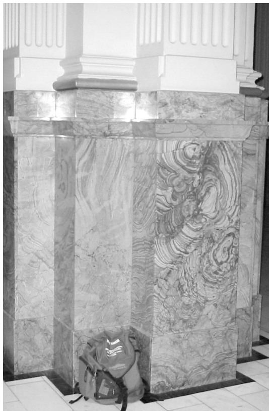
Pillar base at the Colorado State Capitol faced with Beulah Marble from Pueblo County.
