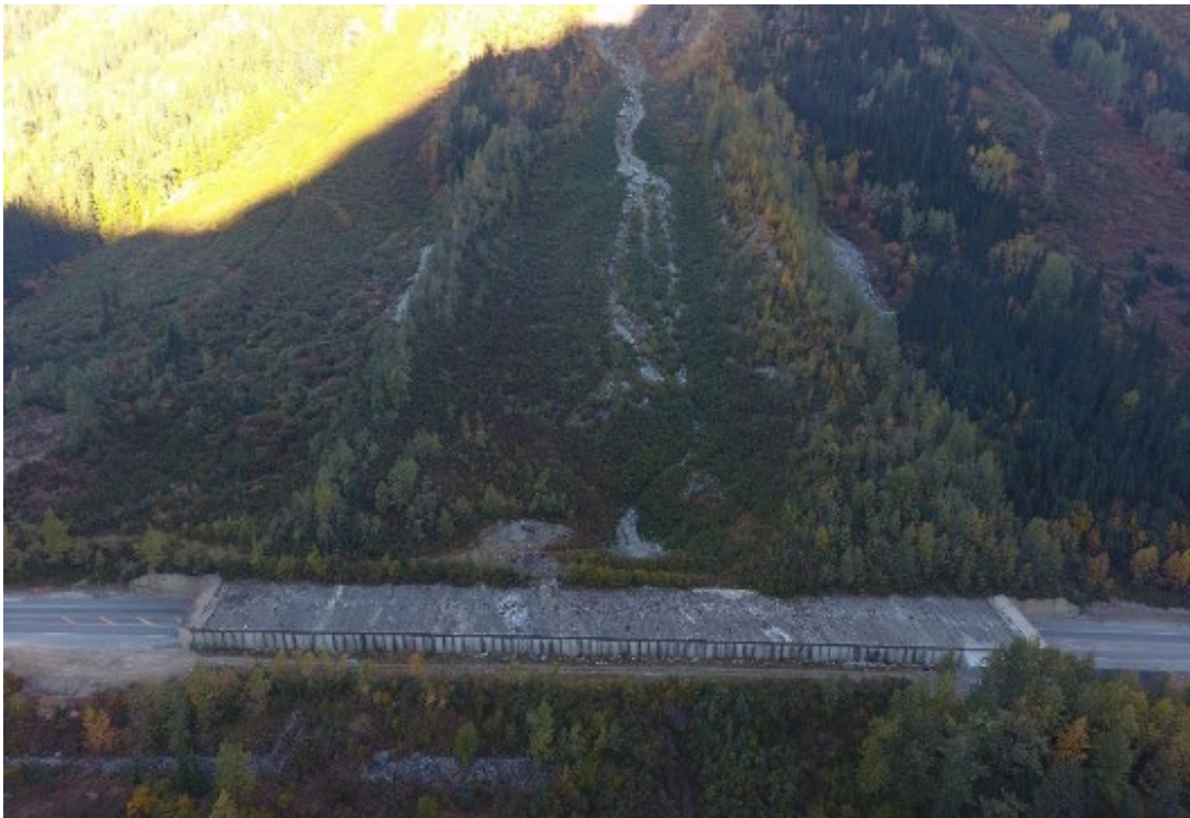
Figure 40: Single Bench avalanche path above the Single Bench snow shed. Single Bench avalanche path is the main path in the center of the photo, directed over the shed and confined by lateral guiding berms. The Mounds avalanche path is immediately west (photo left) of the shed. The Crossover avalanche path affects the shed from the opposite (south) side of the valley, requiring protection of the downslope shed wall (Photo: Dynamic Avalanche Consulting)
