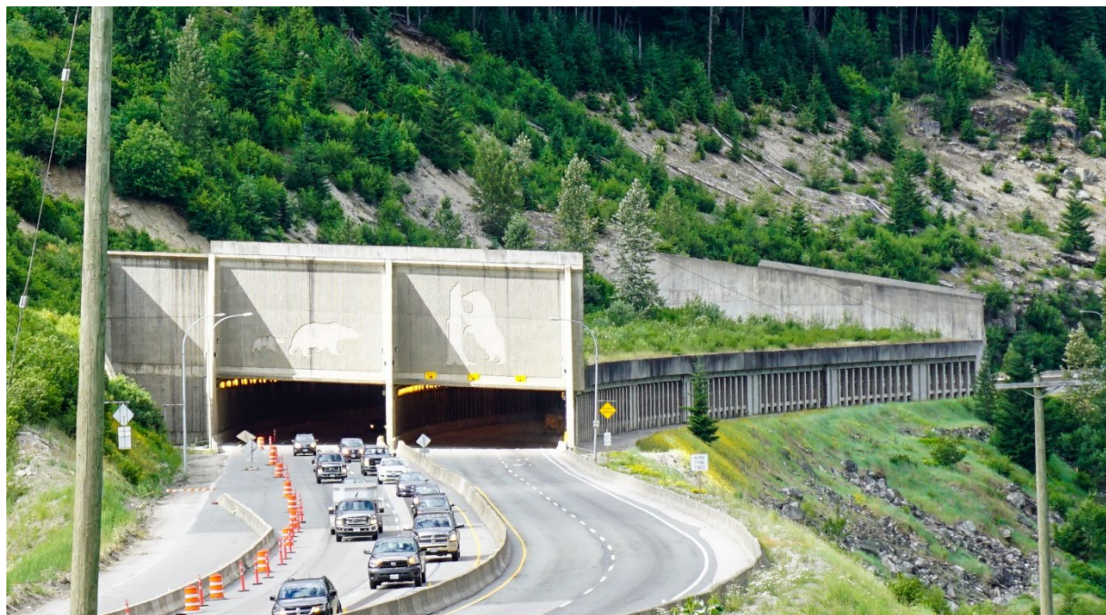
Figure 12: Great Bear snow shed, Coquihalla Highway 5, British Columbia, Canada. Photo is looking eastwards, with steep (8%) grade requiring eastbound trucks to have chains, which increases wear on the roadway surface (and has exposed heat coils). Note the significant horizontal curve which results in super elevation of the highway grade (Photo: Ryan Buhler).
