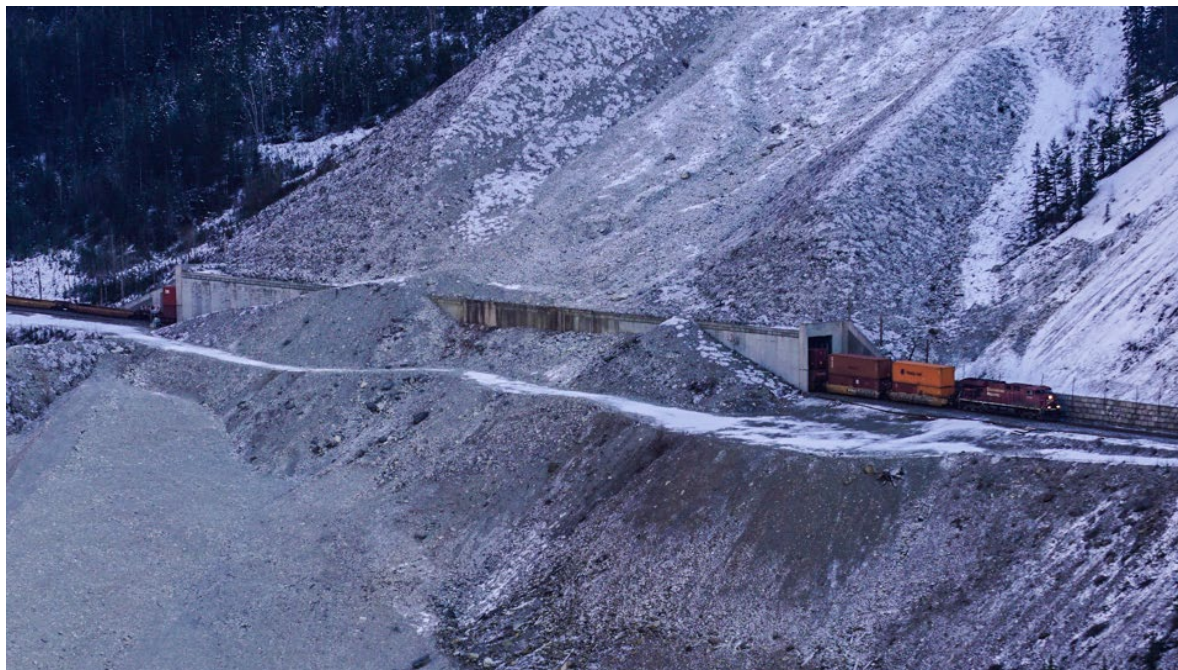
Figure 14: Mt. Stephen snow shed in Yoho National Park, British Columbia, Canada. The shed protects the railway from avalanches, debris flows, and icefall hazards. Avalanches pass over the railway track and affect the highway (Photo: Ryan Buhler).
