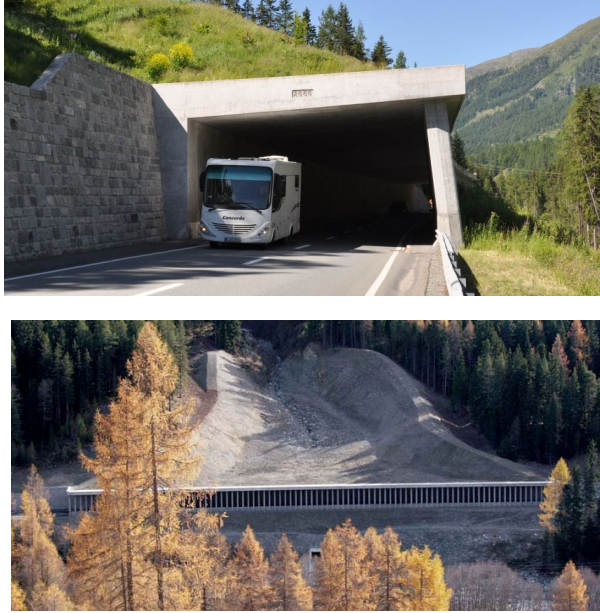
Figure 20: Monolithic Snow shed in Val Raschitsch as viewed from the outside on the side of the road, in profile showing the guiding berms, and the cross section (Photo from Tiefbauamt / Civil Engineering Office Graubünden, Switzerland)
