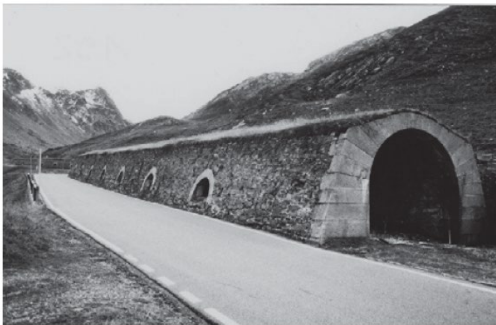
Figure 2: 312m long stone-arched snow shed built at Splügenpass in 1843. The snow shed was in operation until 1950 (Photo: Margreth and Platzer, 2008).
