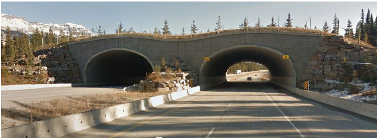
Figure 27: Wildlife overpass on Highway 1 near Lake Louise, Alberta, showing the addition of architectural design elements to the entry, including stacked boulders, trees and vegetation. Similar design elements can be used for snow sheds to enhance the visual appeal and blending in with the natural environment. Photo: Google Maps, 2020.
