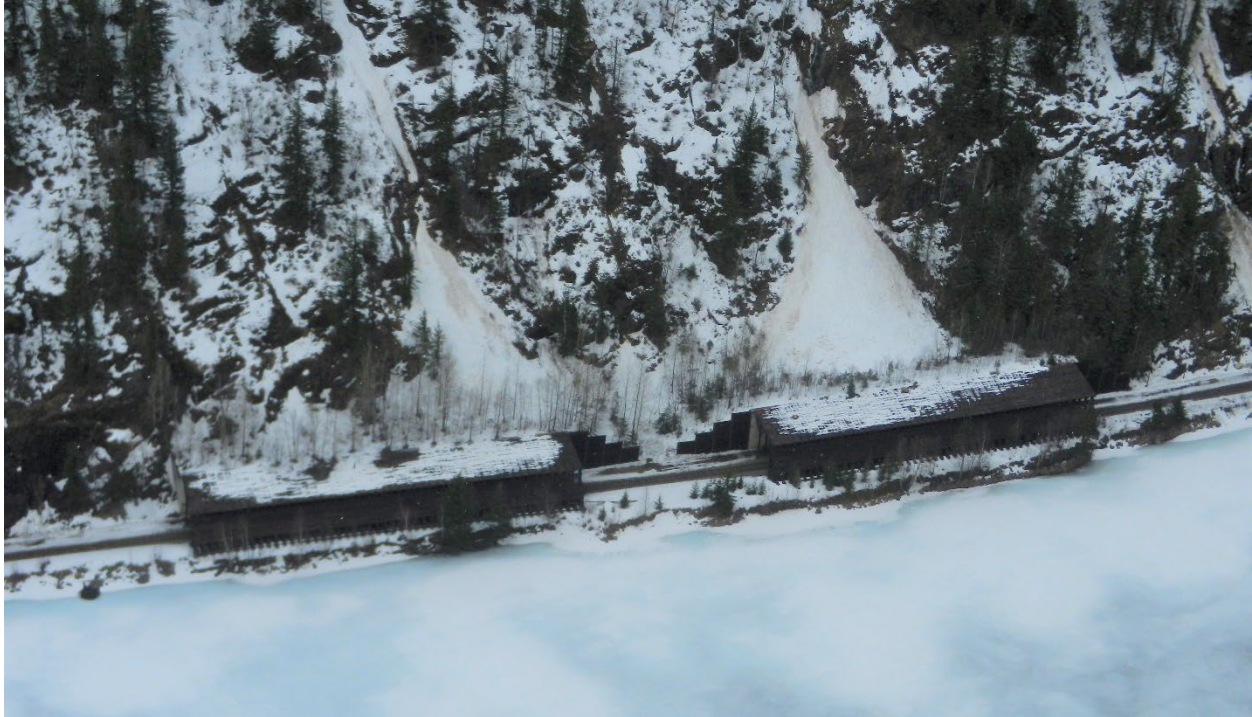
Figure 15: Two wood structure snow sheds that protect the Canadian Pacific Railway at Three Valley Gap near Revelstoke, British Columbia, Canada. Avalanches flow across the shed onto the lake, currently frozen in this photograph (Photo: Alan Jones).
