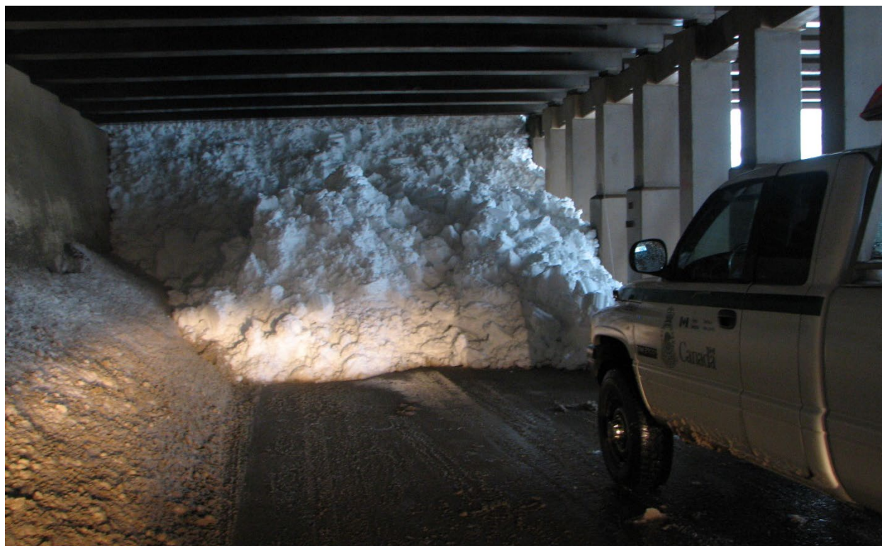
Figure 34: A 2007 overspill in the Tupper #1 snow shed completed blocked the shed portal and caused a lengthy road closure while the deposit was removed.(Photo: Parks Canada).
