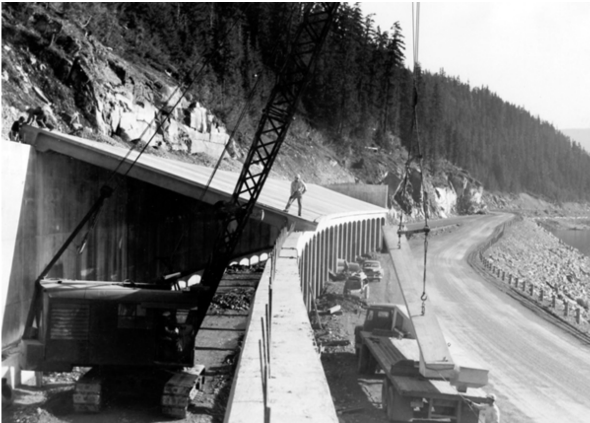
Figure 6: The concrete East Shed was built along Lake Keechelus on I-90 on Snoqualmie Pass in 1950 and now since been removed. (Photo: Washington State Archives 3 )
