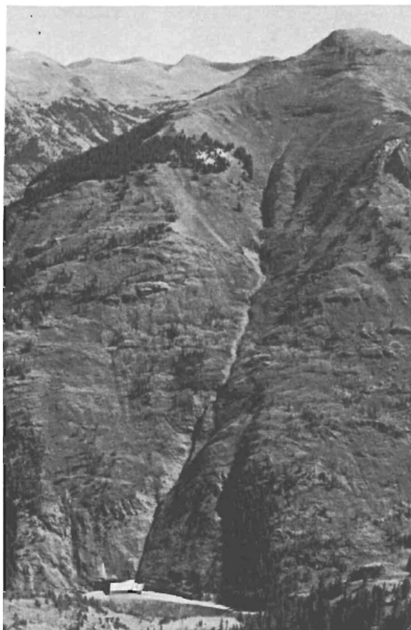
Figure 3: Oblique view of the East Riverside avalanche path and Riverside snow shed (Photo: Mears, 1992).
