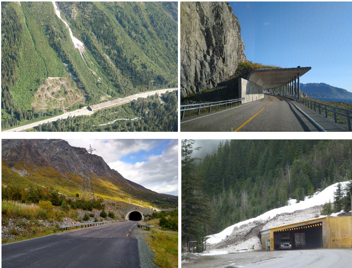
Top left: Single Bench snow shed, BC, Canada (photo: Hendrikk); Top right: Solbjørneset-Hamnøy project, Lofoten, Norway (photo: Hendrikk) Bottom left: Snow shed on Fv91Lyngen, Norway (photo: Hendrikk); Bottom right: Twin snow shed, BC, Canada (photo: Jones)
