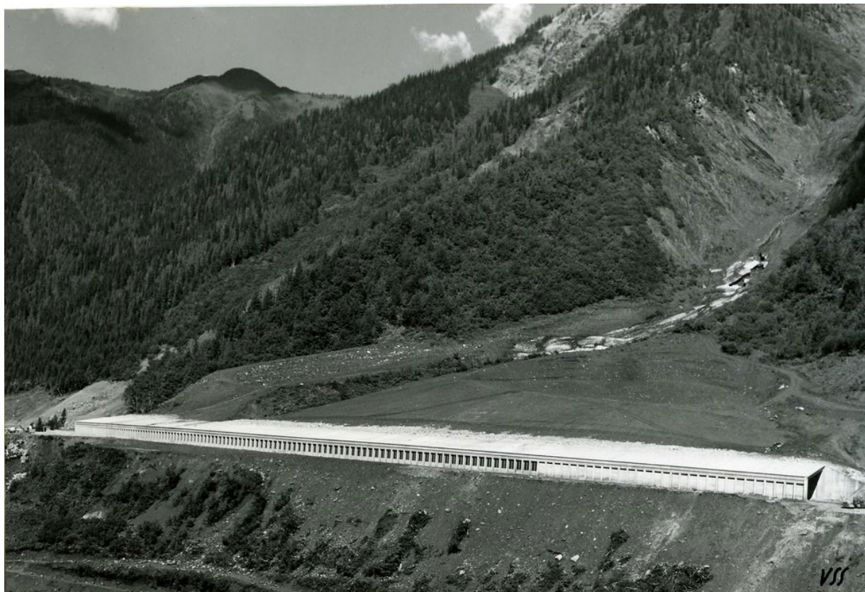
Figure 10: Lanark snow shed built using prefabricated concrete, prior to construction of the wingwalls. Note the guiding berm on the left. (Photo: Peter Schaerer) 6
