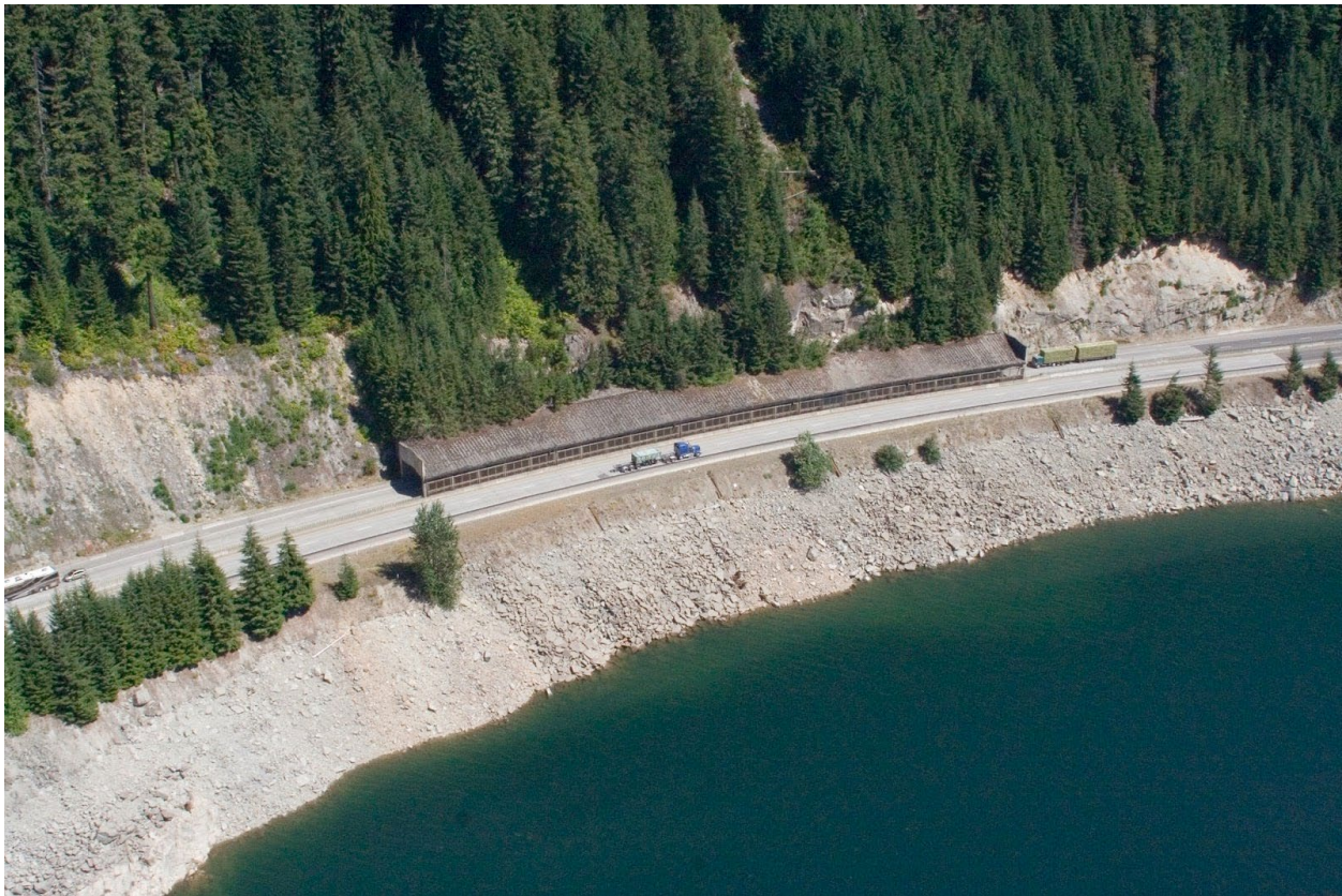
Figure 43: Aerial view of the East Shed in summer prior to its removal, showing the exposed east bound lanes, and covered west bound lanes. (Derrey, 2014)
