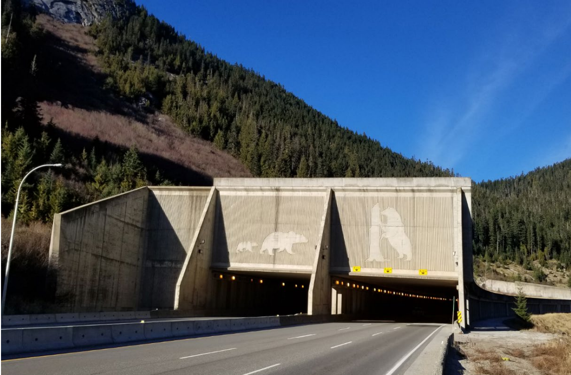
Figure 26: The Great Bear snow shed on the Coquihalla Highway 5, British Columbia, showing the addition of artwork in the concrete wing walls. Photo: R. Buhler.
