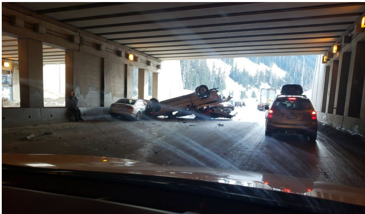
Figure 33: In March 2019, icing in the Great Bear snow shed lead to a five-vehicle collision which sent two people to the hospital (Photo: Global News, 2019) 31 .
