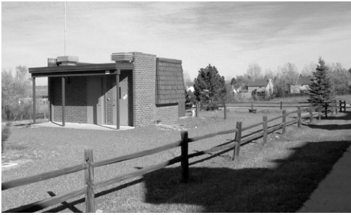
An artificial recharge facility in Highlands Ranch has low visual impact.
