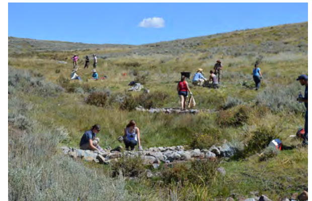
Volunteers building check dams to improve resilience of wet meadows in the Gunnison Basin - a key habitat and source of vulnerability for the Gunnison Sage-grouse.
