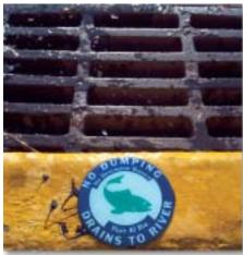
When it rains, dense urban neighborhoods of buildings and pavement create impervious surfaces which don't allow stormwater to infiltrate. Instead, stormwater washes over these surfaces, potentially moving a variety of pollutants into the storm drain system. Water flowing into storm drains (above) is not treated, and may flow directly into rivers and lakes.
