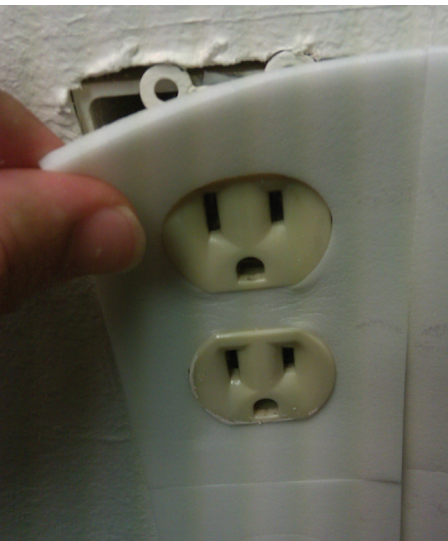
Figure 15. Foam gaskets are an easy fix to air infiltration from electrical outlets on exterior walls.
