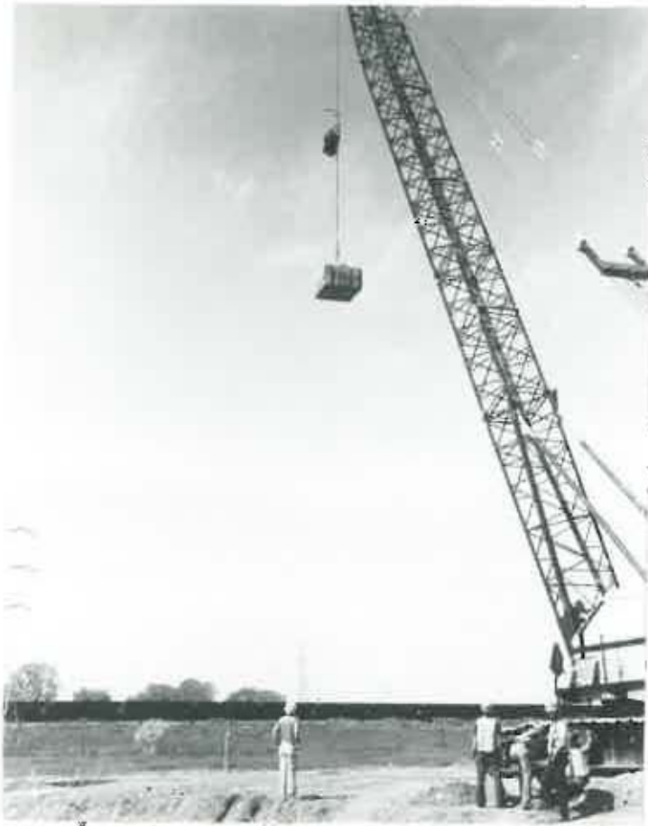
FIGURE 21. CRANE LIFTING THE 20 TON WEIGHT
