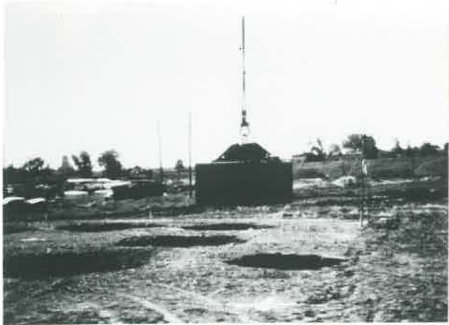
FIGURE 23. CRATERS DURING THE PRIMARY PHASE. THE CRATERS WERE BACKFILLED AFTER COMPLETION OF EACH PHASE
