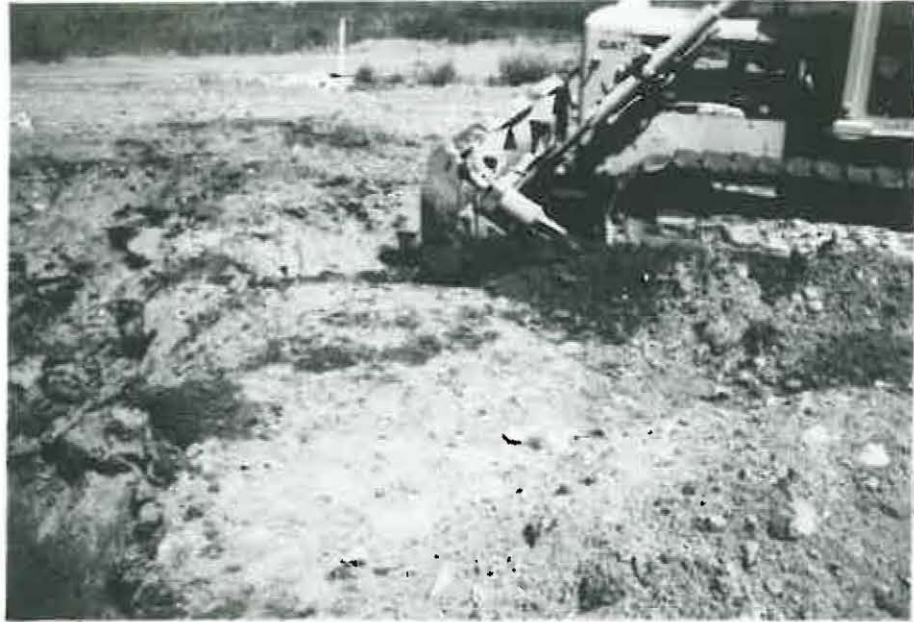
FIGURE 25. CRATERS WERE BACKFILLED WITH GRANULAR MATERIAL
