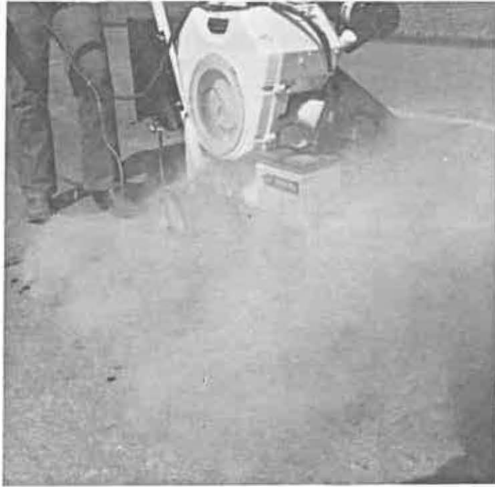
This machine is a short pivotal saw used to rout cracks.
