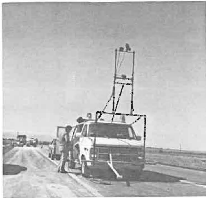
Non-destructive testing (NDT) equipment used on the preliminary engineering condition survey. Donahue Radar Void Detector which was one of several pieces of NDT equipment on display at the project site. This device is used to detect voids under the faulted slabs.
