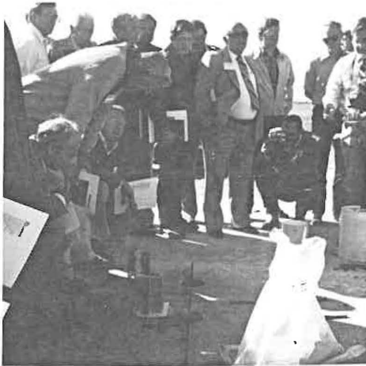
A group of attendees watching a demonstration on installing the load transfer devices.
