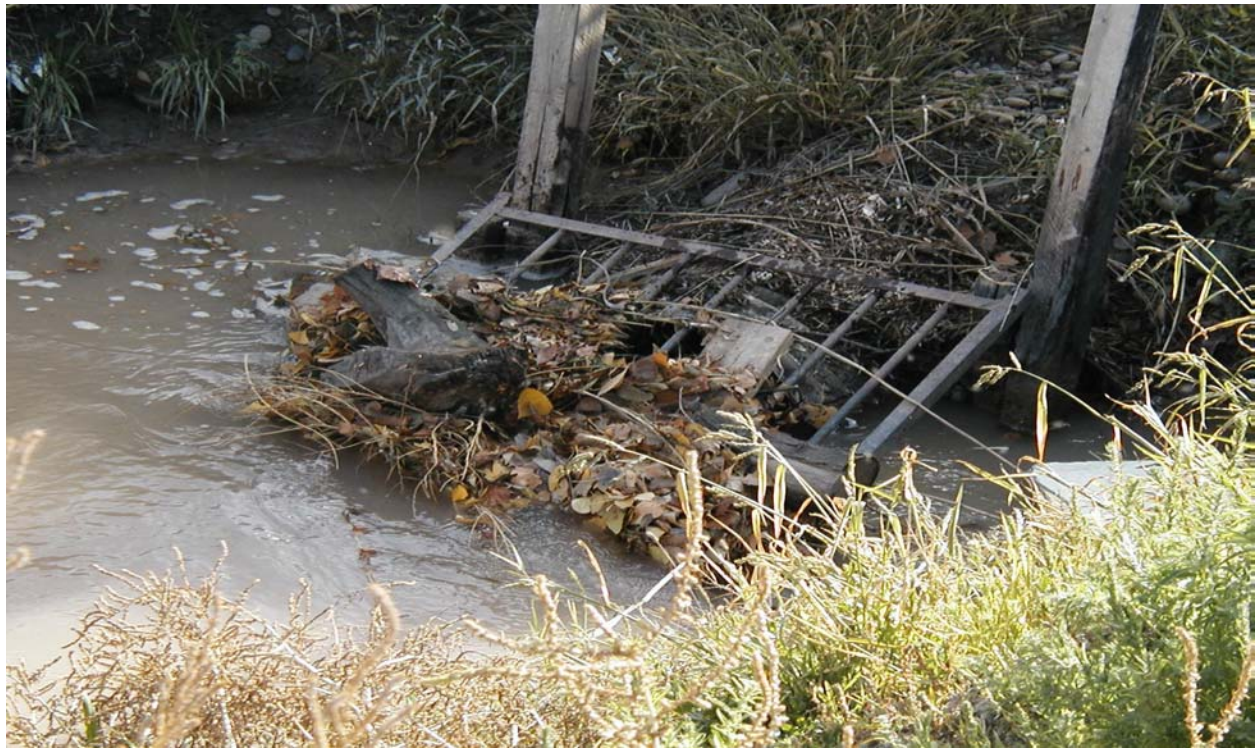
Figure 3. Example of Common Maintenance Needs
