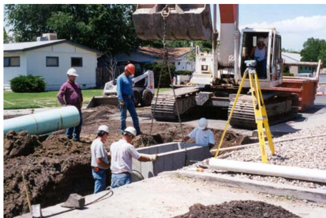
Orchard Avenue Major Storm Sewer Construction, Summer 1999
