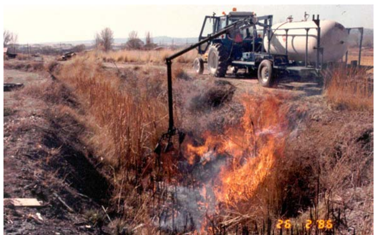
Burning Vegetation to Reduce Fire Danger, Maintain Capacity and Clean Ditch
