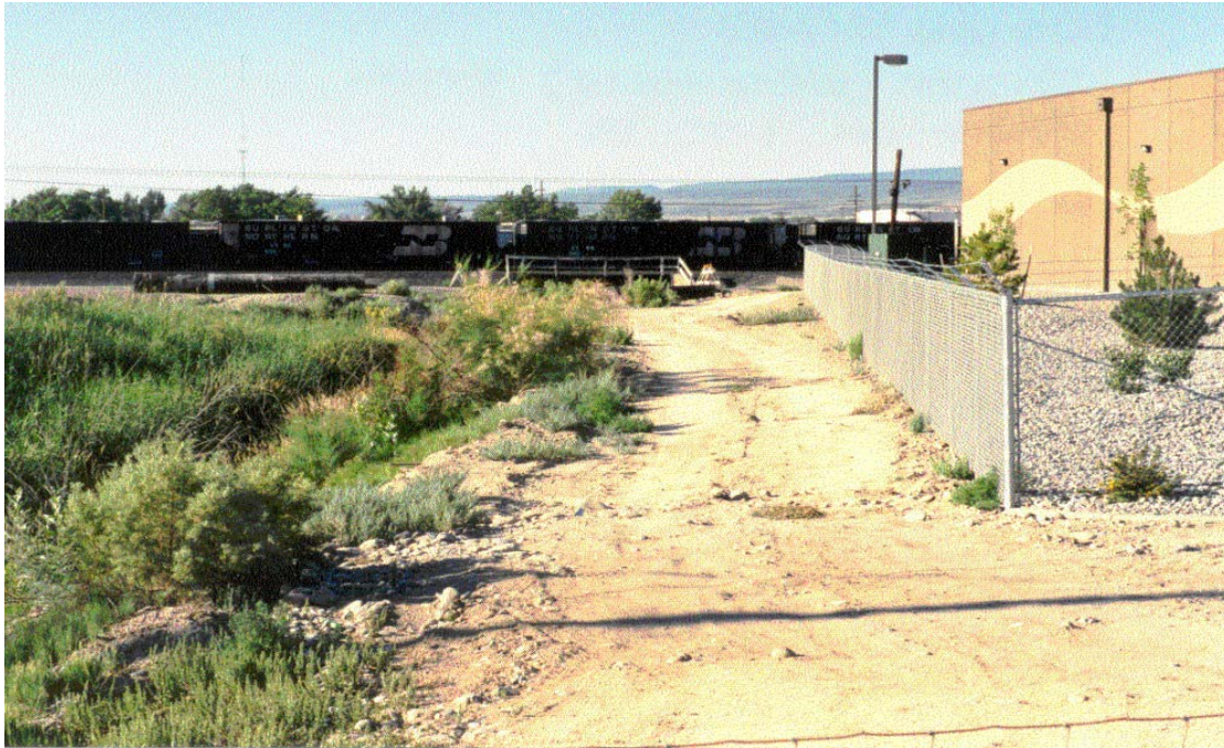
Figure 7. Hindrances to Maintenance Access
