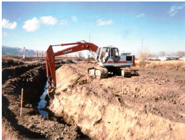
Ligrani Drain - Typical Open Drain Maintenance Activities
