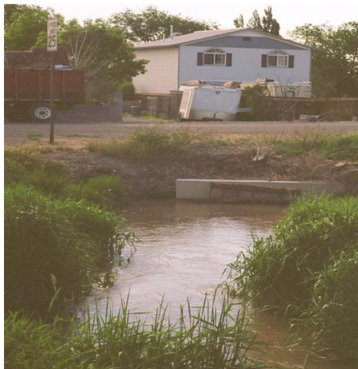
Figure 12. Orchard Mesa Drain Full of Irrigation Water, May 2003 Palisade Street South of Unaweep (No available capacity for stormwater)
