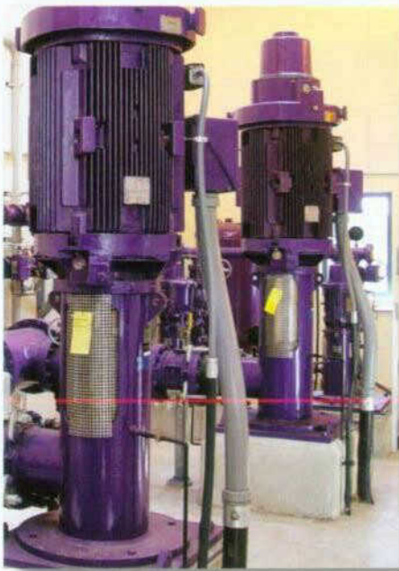
Reuse of nonpotable water for commercial and industrial uses, such as irrigation of golf courses or industrial cooling, is becoming increasingly common in Colorado and the West. Pipes and machinery used for nonpotable water are colored purple to distinguish them from drinking water and sewer lines.
