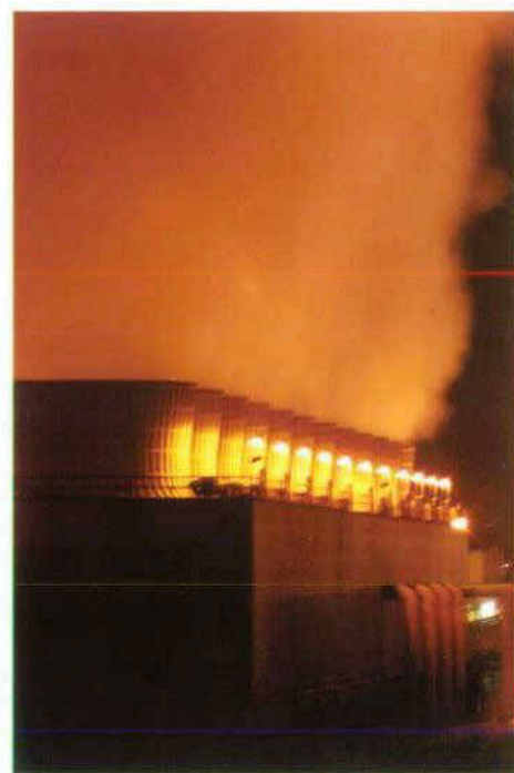
Cooling towers, such as these owned by Xcel Energy, consume large quantities of water through evaporation.
