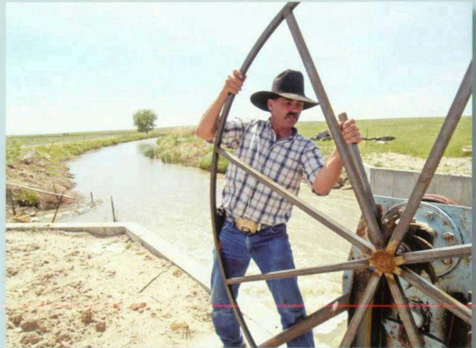
Dan Henrichs, superintendent of the High Line Canal, adjusts one of the gates that helps meter the canal's flow to farm fields and ranch pastures throughout the Lower Arkansas River Valley.
