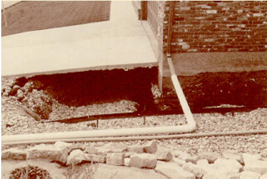
Figure 10. Cross section and photograph of a subsidence pit, under a house, in an area of thick soil cover. (P.B. DuMontelle, 1981, *Mine Subsidence in Illinois: Facts for the Homeowner*, I.G.S., Environ. Note 99. (photo by L. Floyd, Office of Surface Mining))
