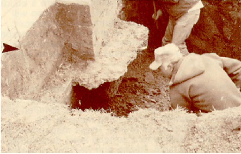
Figure 19. A subsidence pit formed under the corner of this house. The structure was able to span the void with minor structural damage. (*photo courtesy of L. Floyd, Office of Surface Mining*)
