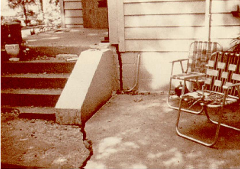
Figure 22. Tensional forces caused the steps and porch of this house to pull away from the main structure. (*photo courtesy of Colorado Mined land Reclamation Division*)
