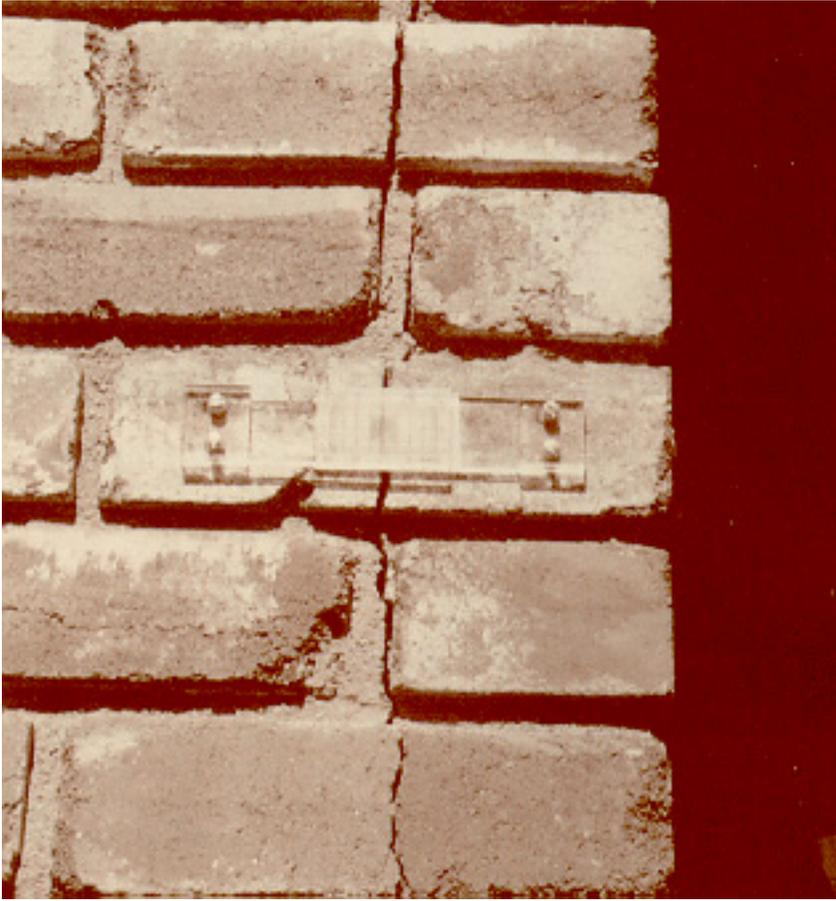
Figure 28. Tension fracture in brick. A fixed monitoring grid covers the fracture. Note how the fracture cuts the brick. (*photo courtesy of L. Floyd, Office of Surface Mining*)
