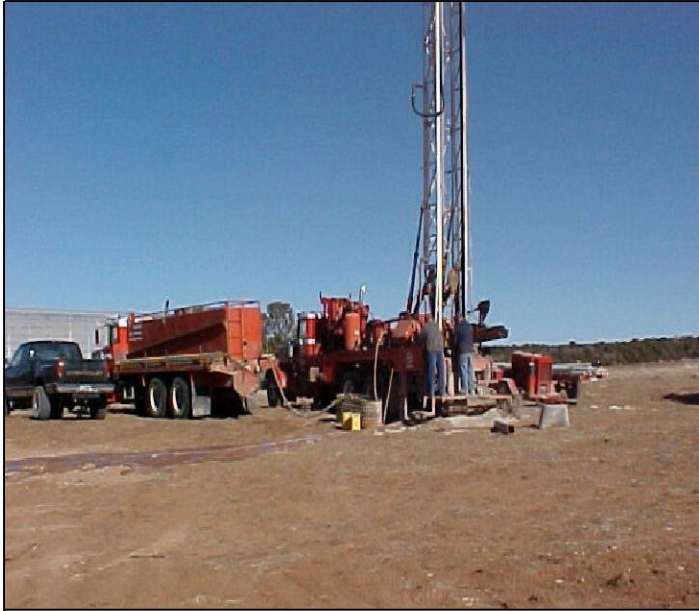
Drilling and support vehicles
