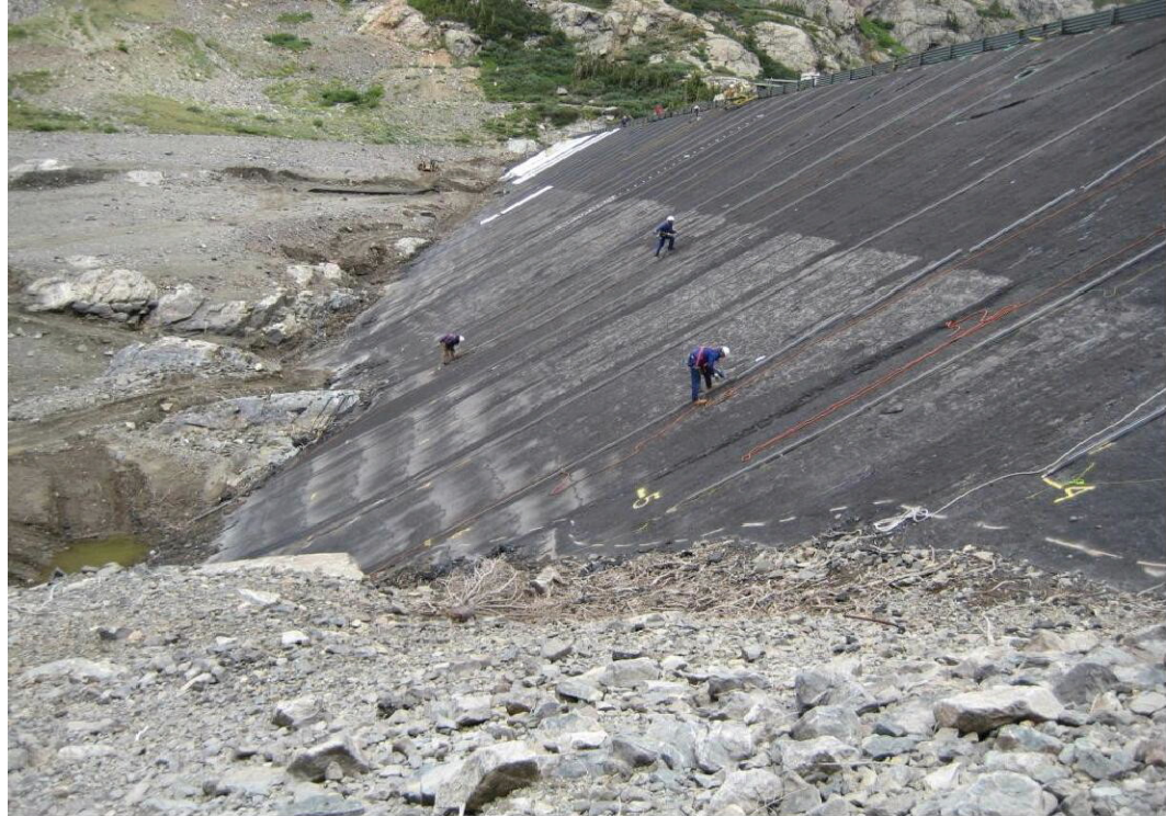
Upper Blue Dam, Summit County, Division 5. High Hazard
