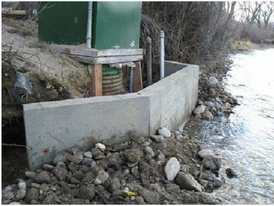
Arkansas River at Salida flood wall
