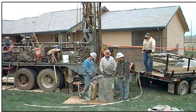
Plugging and abandoning a well in the Laramie-Fox Hills aquifer
