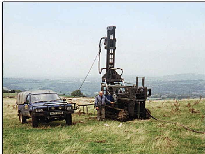
A homemade drill rig at an unknown location
