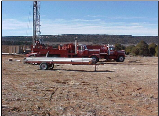
Drill rig and casing trailer at a new residential building site.
