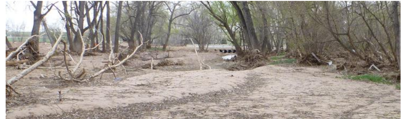
Looking downstream at temporary culverts placed at 83rd Street
