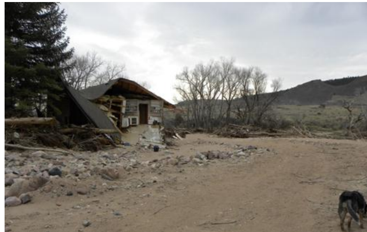
Residence downstream of Stagecoach Trail
