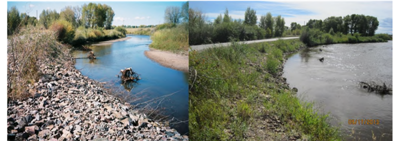
Rootwad revetment with scour toe protection and vegetated bank stabilization, Laramie, WY
