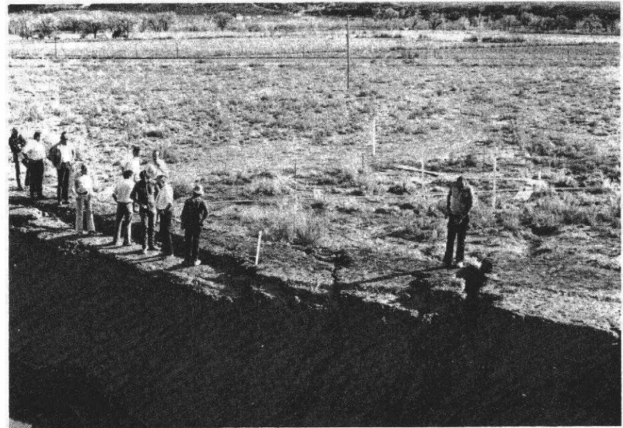
Tests permitted proper highway design and construction, avoiding future repairs.
