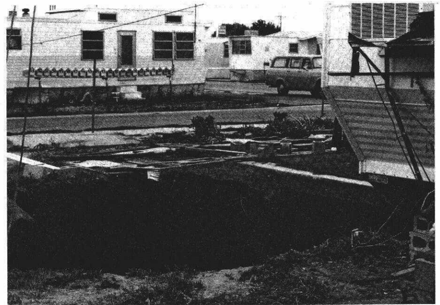
Subsidence pit in a trailer park at Lafayette. This 25 ft x 25 ft hole, 30 ft deep resulted from collapse of the overlying materials into an inclined mine shaft.
