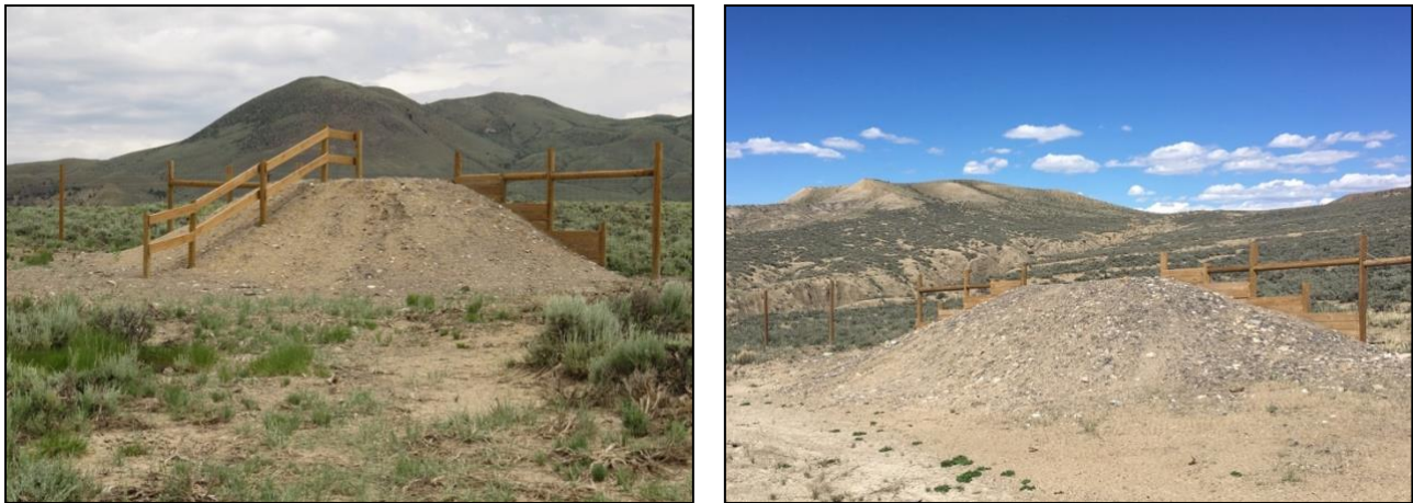
Figure A-2. Example of an escape ramp with a 2:1 slope with perpendicular rail fence (left) and a ramp with a 3:1 slope with no rail fence (right).
