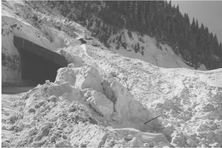
The avalanche shed saves lives and keeps the highway open.
