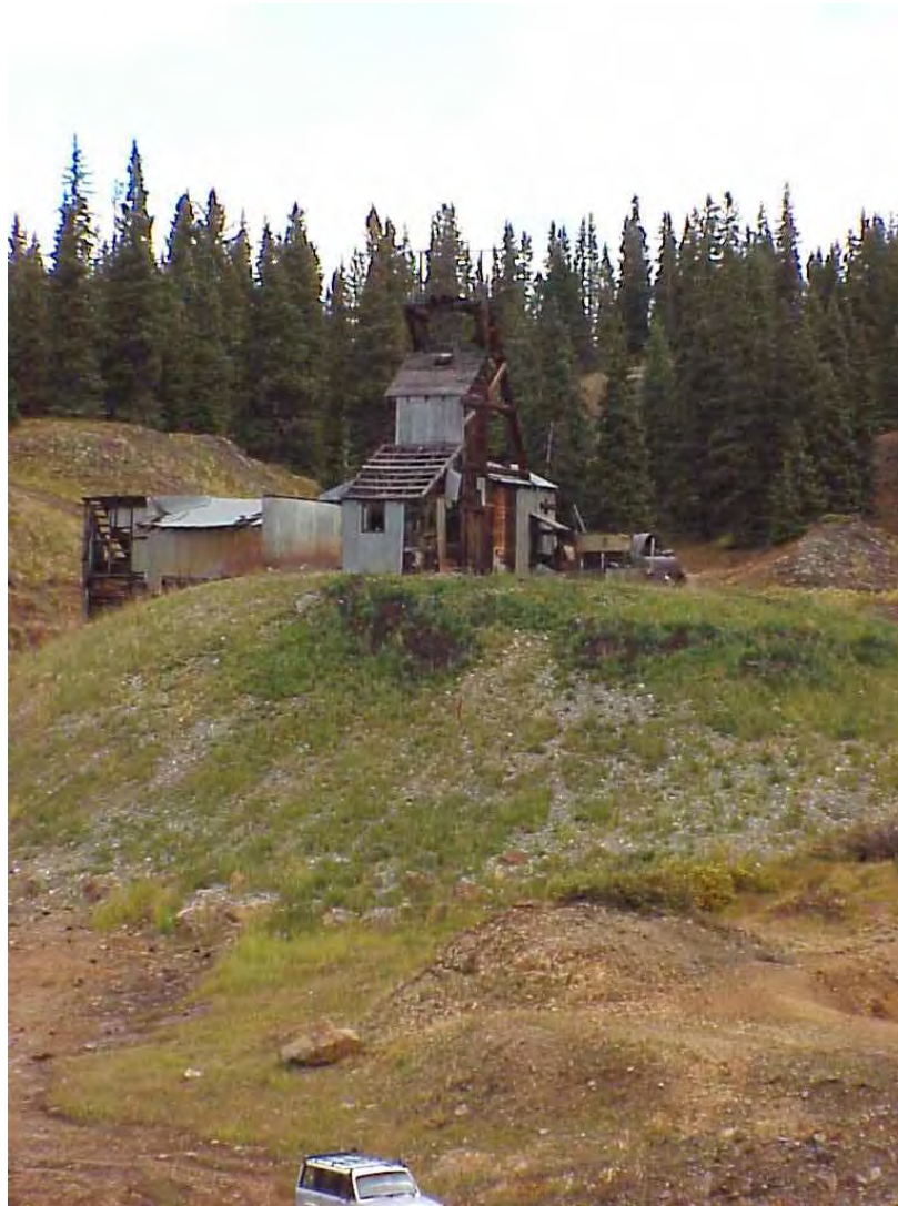
Longfellow Mine shaft house. The waste-rock dump around this mine has undergone reclamation. (Stop 5)
