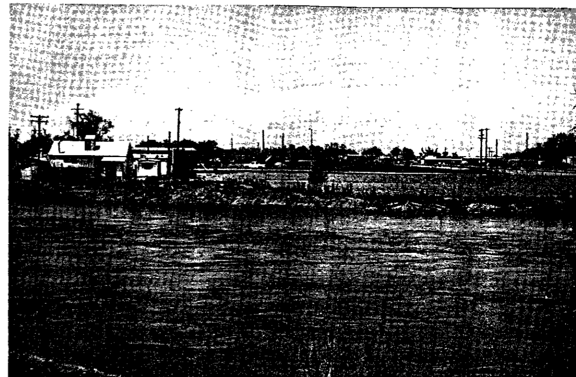
LOOKING NORTHEAST BETWEEN 8TH. STREET AND U.S. 85 BYPASS
