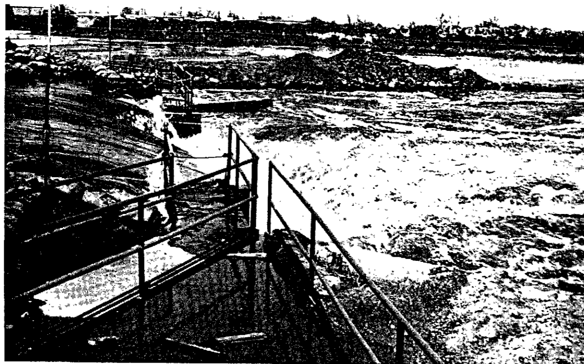
CONTROL STRUCTURE AT WASTEWATER TREATMENT PLANT
