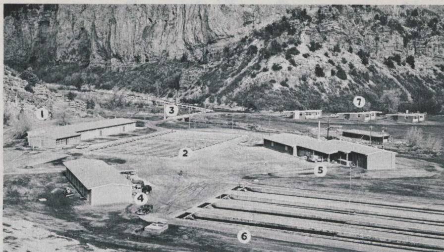
Rifle Falls is the department's largest unit. Shown are (1) hatchery, (2) nurse ponds, (3) water source, (4) garage, (5) feed storage building, (6) raceways, (7) housing.
