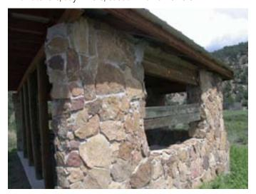
BLIND DESIGN/ CONSTRUCTION Design: Natural stone with timber roof framing
