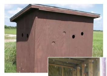
Materials: Treated 2x4's and plywood, with painted exterior.
