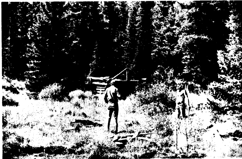
Fig. 14. An old miner's cabin near the headwaters of the Blue River is being dismantled by an individual who stated he was working for a local contractor who wanted the old lumber to provide a decorative atmosphere to condominiums. Note pile of wood in foreground.
