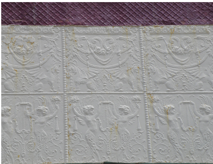
Pressed tin cornice
