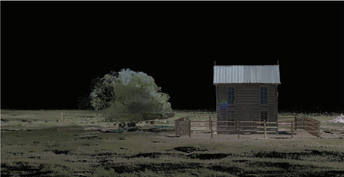
Front view of Pedro Trujillo two-story log cabin
