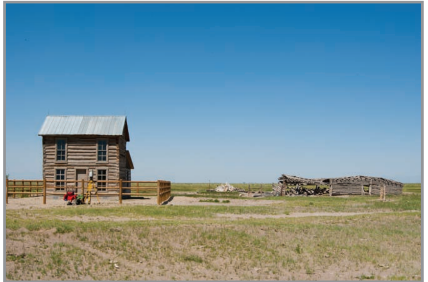
View of Pedro Trujillo house and stable with scanner in the foreground
