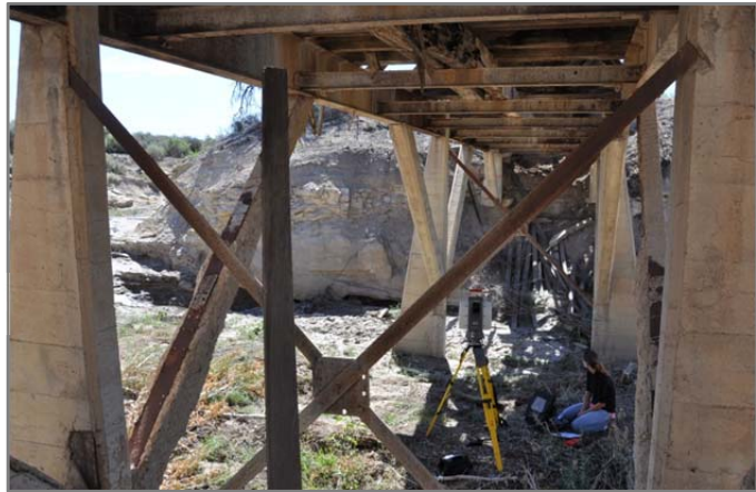
McElmo Flume being scanned by Leica Scan Station 2
