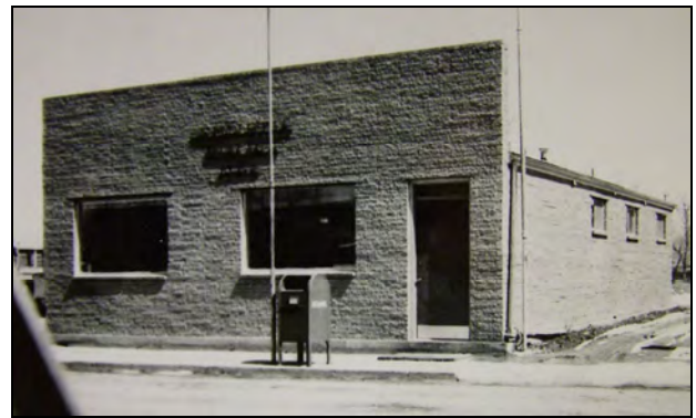
Figure 21. The 1961 Genoa U.S. Post Office reflects Modern influences. SOURCE: Lincoln County Assessor, old appraisal card photograph, 1970.
