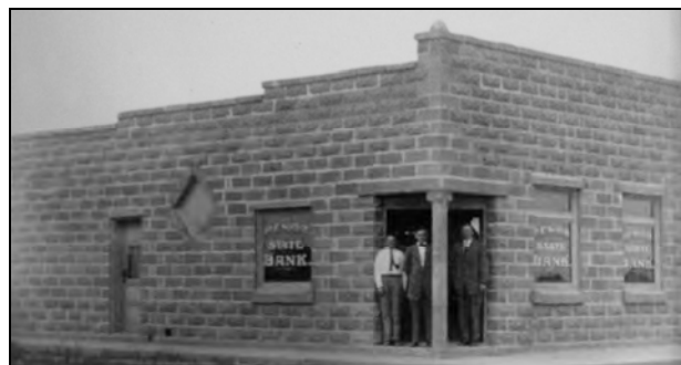
Figure 8. The Genoa State Bank, which opened its doors in early 1910, was built of ornamental concrete blocks. SOURCE: Hedlund House Museum, photographic collection, Hugo, Colorado.
