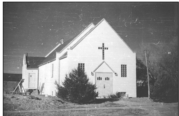
Figure 16. Trinity Evangelical Lutheran Church was completed in 1948. SOURCE: Hedlund House Museum, photographic collection, Hugo, Colorado.
