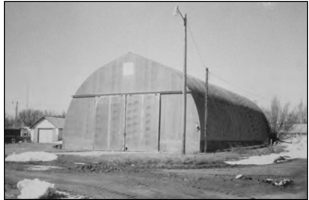
Figure 23. The DaVatz Quonset is an example of the pointed arch variety. SOURCE: Lincoln County Assessor, old appraisal card photograph, 1987.
