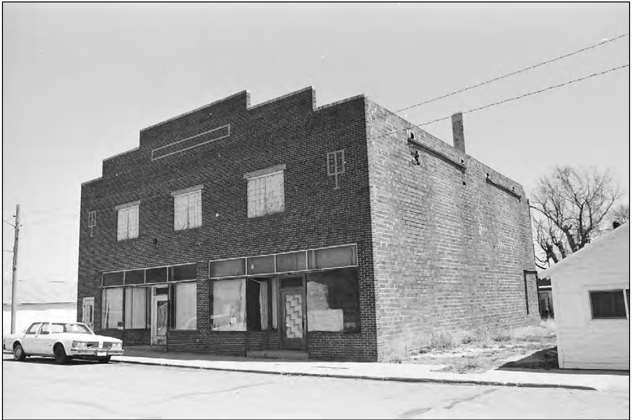
Figure 24. The brick and hollow clay block Hunt Building at 301 Main Street is Genoa's only two-story commercial building. SOURCE: Thomas H. Simmons, fieldwork photograph, April 2008.
