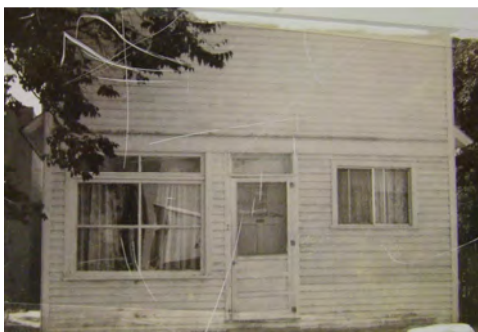
Unknown (between 1970 and 1988). The north storefront window has been replaced but the false front is still present.
