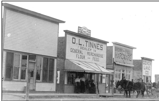
Figure 7. False front buildings, such as these on the west side of Main Street (400 block), were a common sight during the early settlement period in towns throughout Colorado. SOURCE: Hedlund House Museum, photographic collection, c. 1908, Hugo, Colorado.
