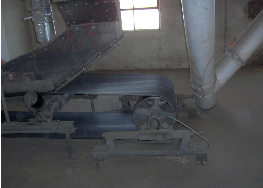
Figure 6: Terminal Elevator Conveyor, Paoli, Colorado, University of Colorado Denver
