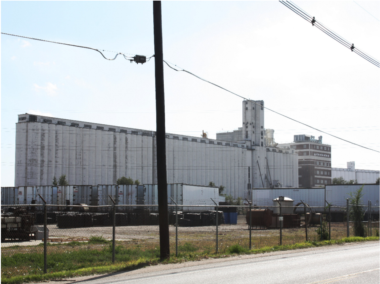
Figure 26: Corporate Elevator, Commerce City Grain/ Conagra Foods, Commerce City, Colorado, University of Colorado Denver. The Colorado Milling and Elevator Company was a predecessor to Conagra.
