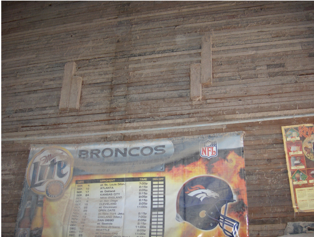
Figure 8: Interior Cribbed Elevator, La Junta, Colorado, University of Colorado Denver
