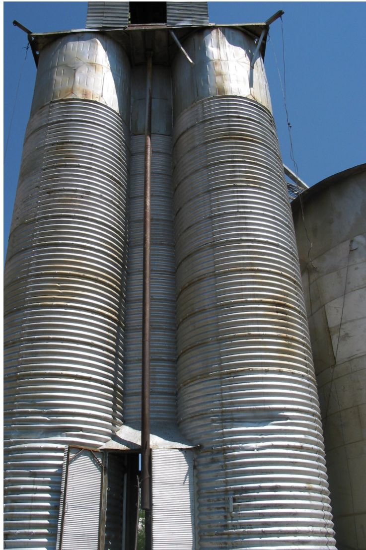
Figure 12: Steel Bin Elevator, Kit Carson, Colorado, University of Colorado Denver
