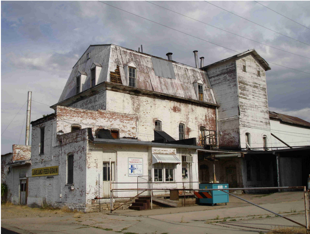
Figure 18: Loveland Mill, Brick Construction, Loveland, Colorado, University of Colorado Denver
