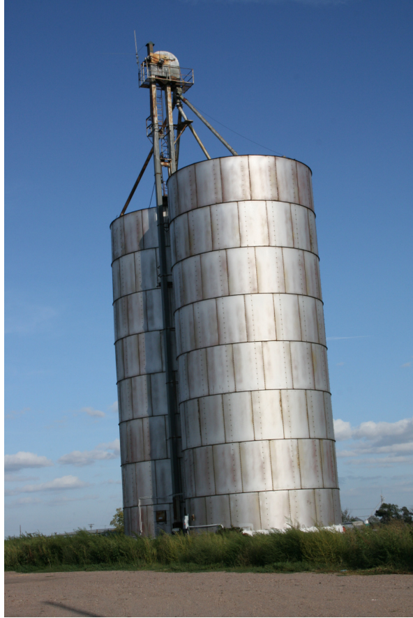
Figure 13: Steel Tile Elevator with Open Leg, Cheyenne Wells, Colorado, University of Colorado Denver
