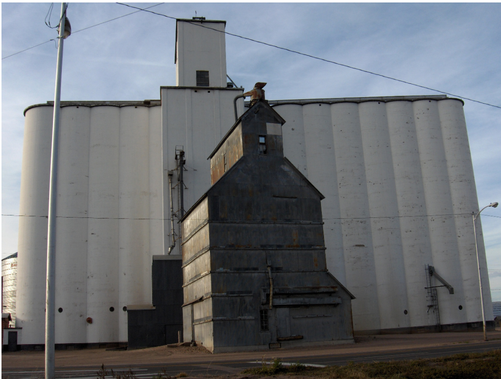
Figure 2: Country and Terminal Grain Elevators, Julesburg, Colorado, University of Colorado Denver
