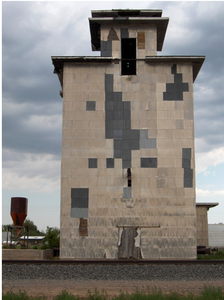
Figure 7: Cribbed Elevator, Campo, Colorado, University of Colorado Denver
