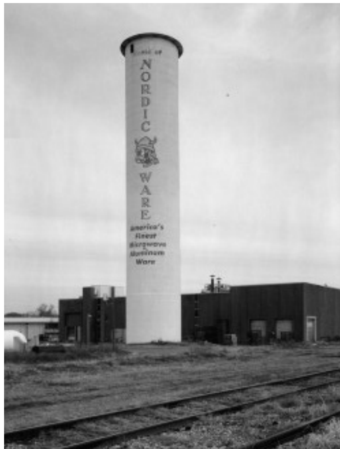
Figure 15: Peavy-Haglin Experimental Concrete Elevator, St. Louis Park, Minnesota (HAER)
