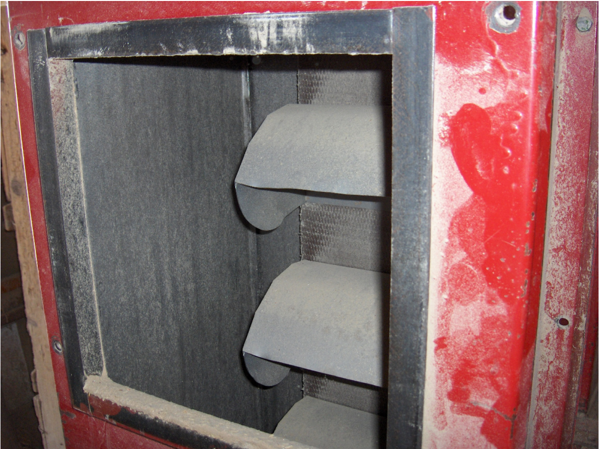
Figure 4: Country Grain Elevator Leg, La Junta, Colorado University of Colorado Denver
