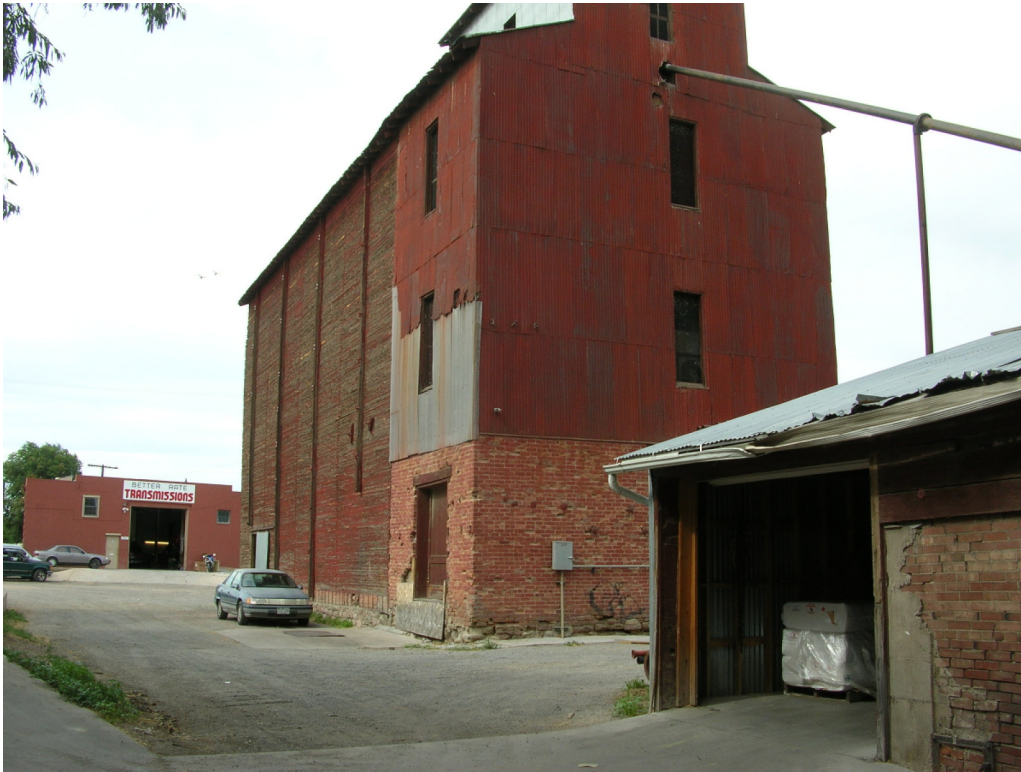
Figure 20: Pueblo Flour Mill, Pueblo, Colorado, University of Colorado Denver
