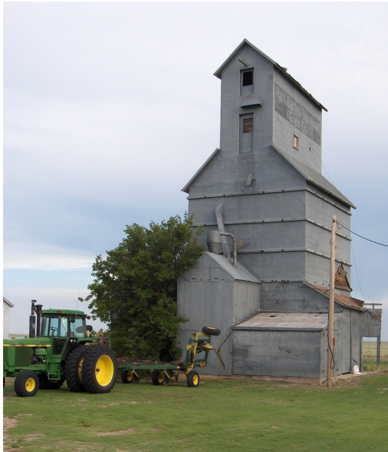
Figure 9: Stud Elevator, Pritchett, Colorado, University of Colorado Denver
