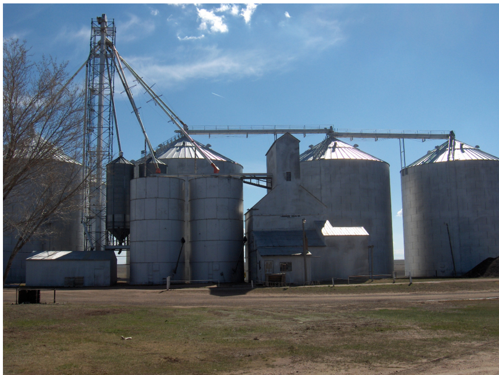
Figure 10: Expanded Wood Elevator, Raymer, Colorado, University of Colorado Denver
