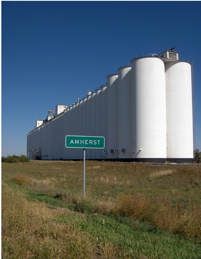
Figure 17: Concrete In-land Terminal Elevator, Amherst, Colorado, University of Colorado Denver
