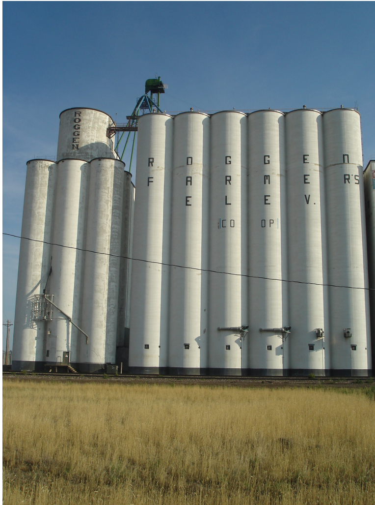
Figure 27: Roggen Elevator Co-op, Roggen, Colorado, University of Colorado Denver. The image is typical of the concrete Farmer's Cooperative Elevators across the Eastern Plains.
