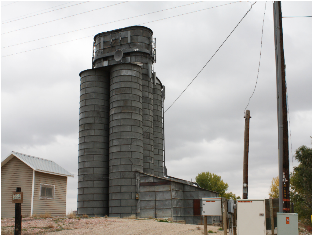
Figure 11: Steel Tile Elevator, County Road 20, Larimer County, University of Colorado Denver
