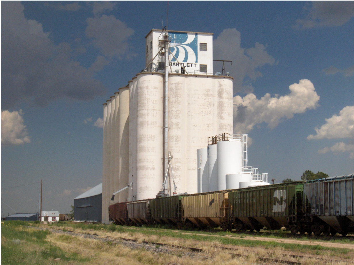
Figure 25: Line Elevator, Bartlett Grain Company, Walsh, Colorado, University of Colorado Denver
