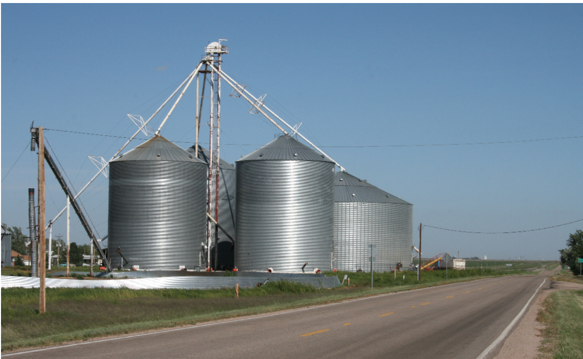
Figure 14: Steel Silo Feed Handling Center, Bethune, Colorado, University of Colorado Denver
