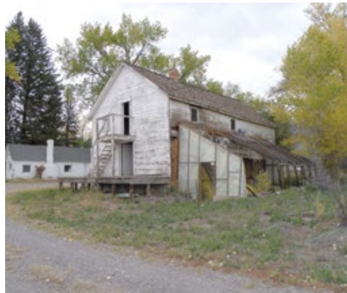
Feed and seed storage building with office/ bunkhouse behind.
