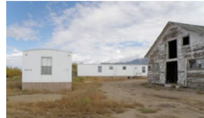
View of storage building and the two newest trailers on site.
