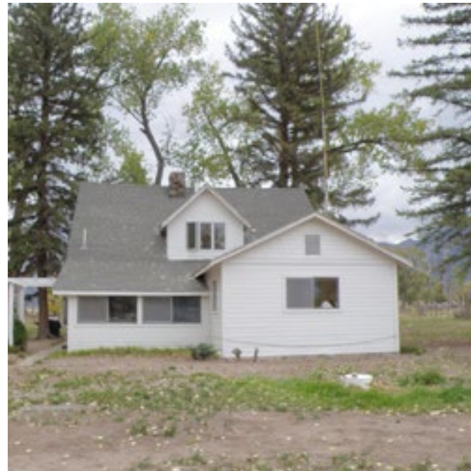
View of the headquarters/ office.
