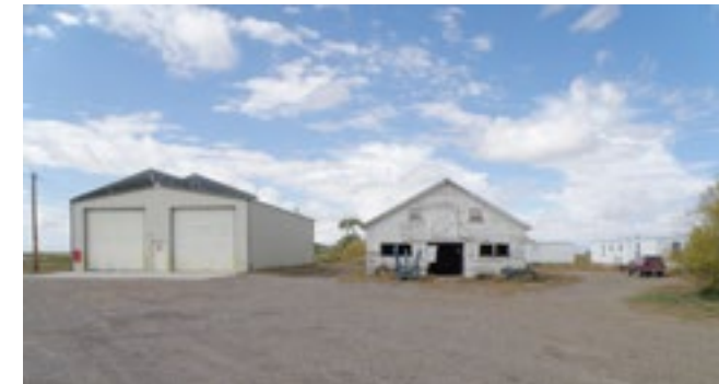
View of storage building and metal building with trailers in the background.
