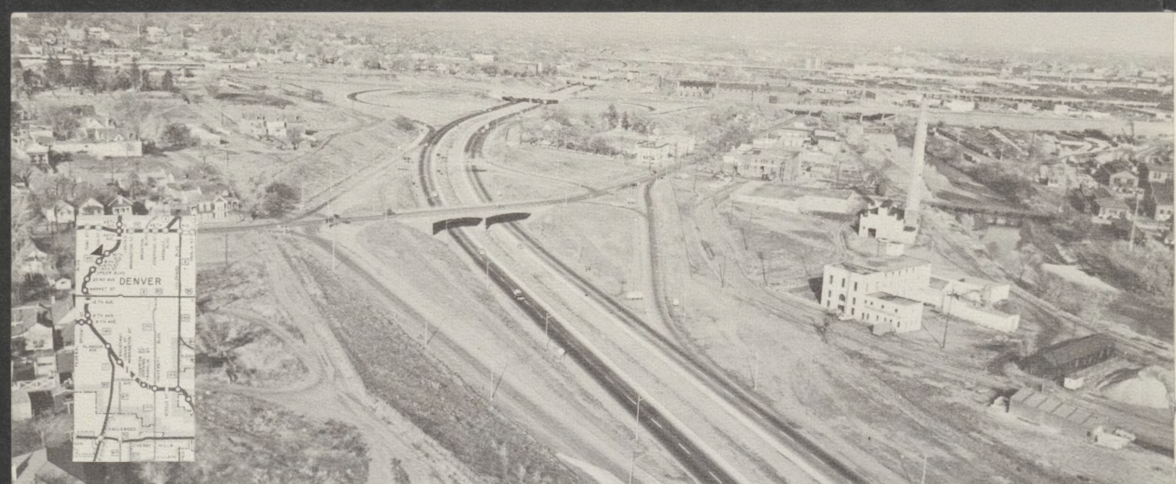
THE WEST 23RD AVE. INTERCHANGE, which you just entered from the last picture. This interchange is what is known as the "Diamond" type. It may be compared with the cloverleaf
