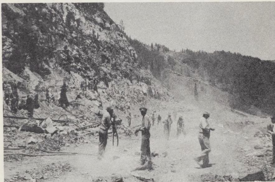
Drilling holes for blasting on Coalbank Hill job on U.S. 550.
