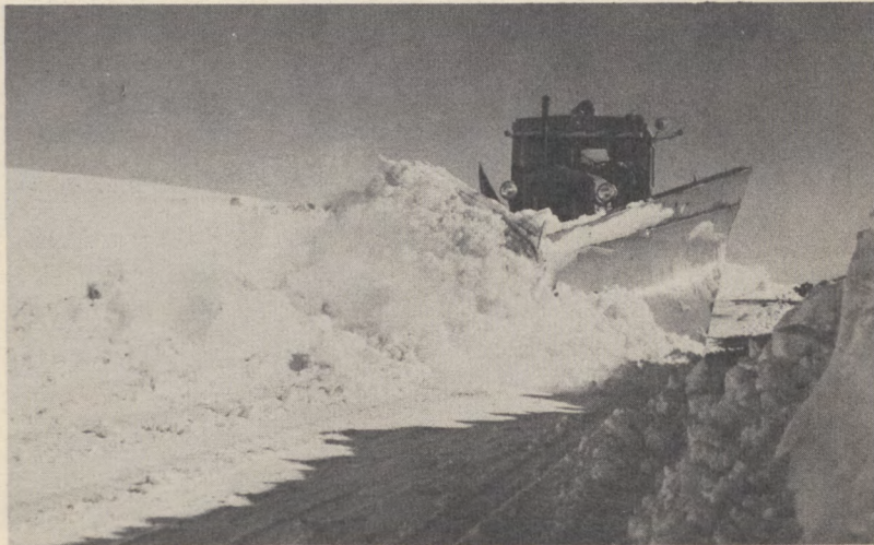
"A" plows (named from their shape) smash open big drifts
