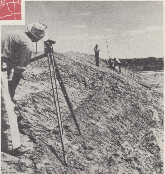
Survey parties lay line of a smooth road over uneven terrain.
