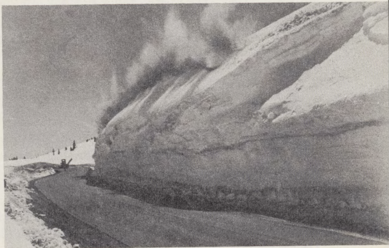
Dynamite charges are here about to shear off a cornice.
