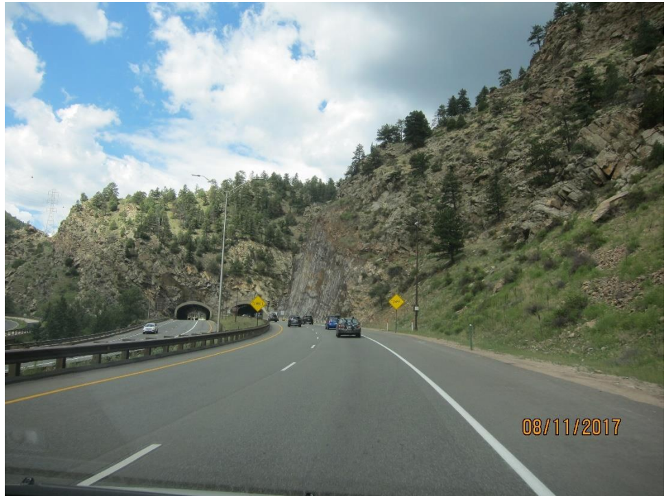
Looking west at approximately MP 242.
