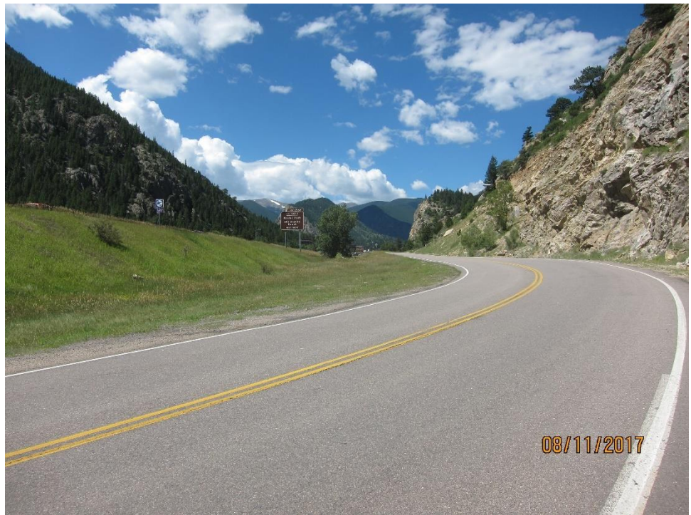
CR 308 adjacent to the north of I-70 at MP 233.
