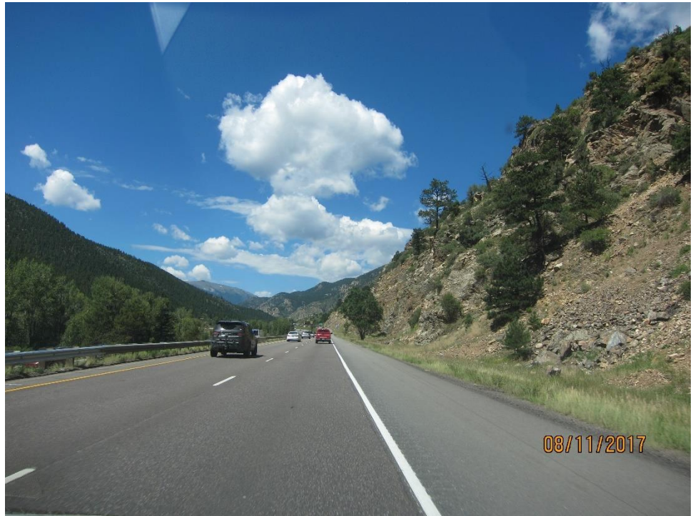
Looking west along I-70, approximately at MP 236.
