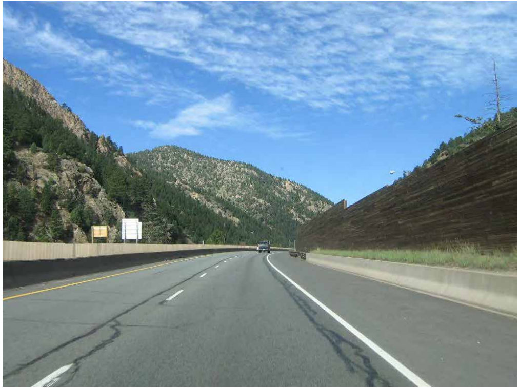
Photo 9. View of I-70 looking west.
