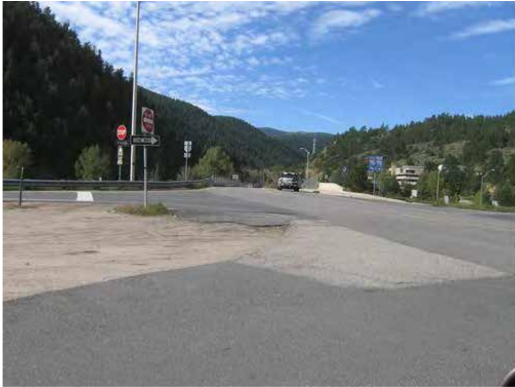
Photo 7. View of structure F-14-E, bridge carrying SH-103 over I-70. Bridge will be replaced during project activities.
