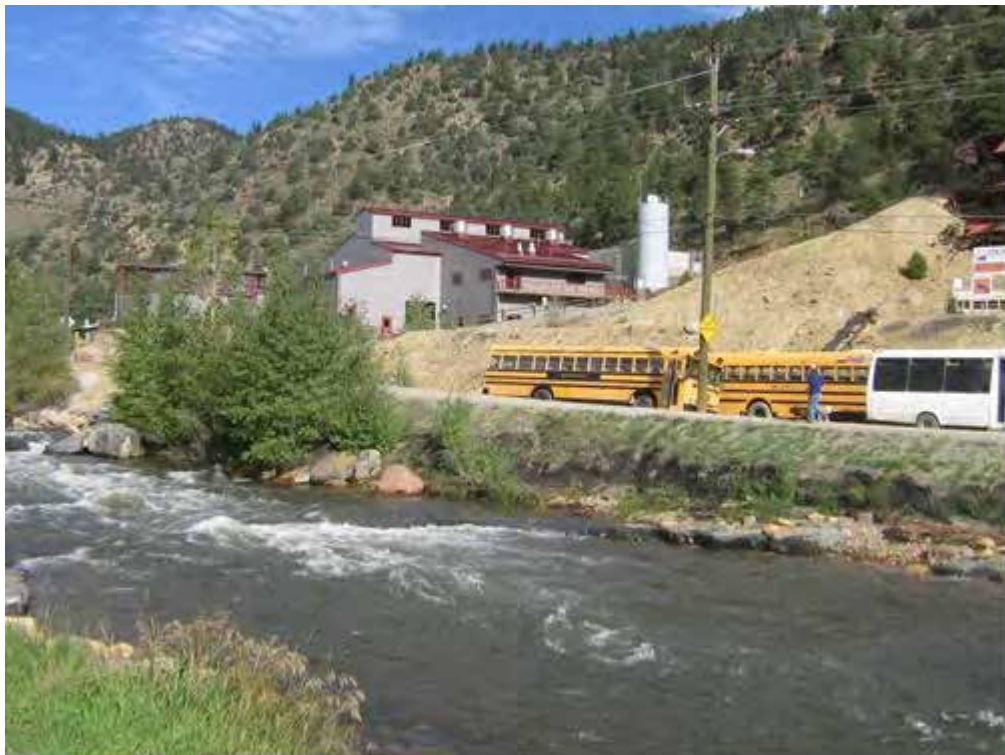
Photo 2. View of Argo Water Treatment Facility and Clear Creek.
