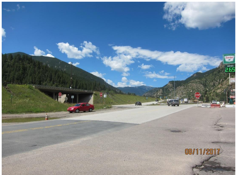
Overpass and truck scales at I-70 exit 234.
