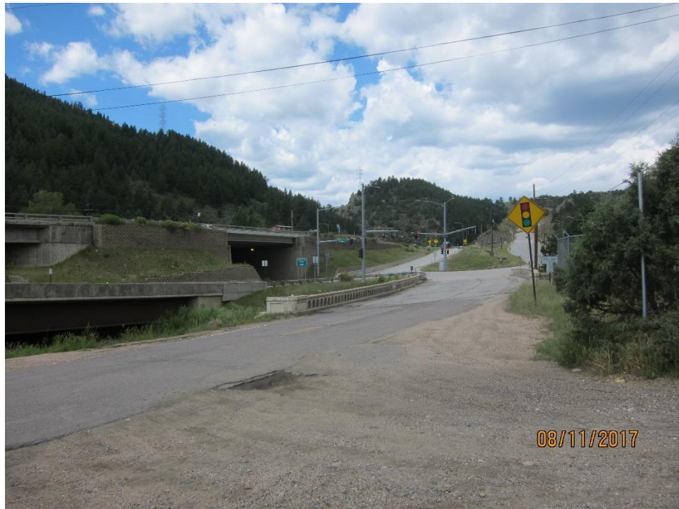
Overpass at I-70 exit 243.
