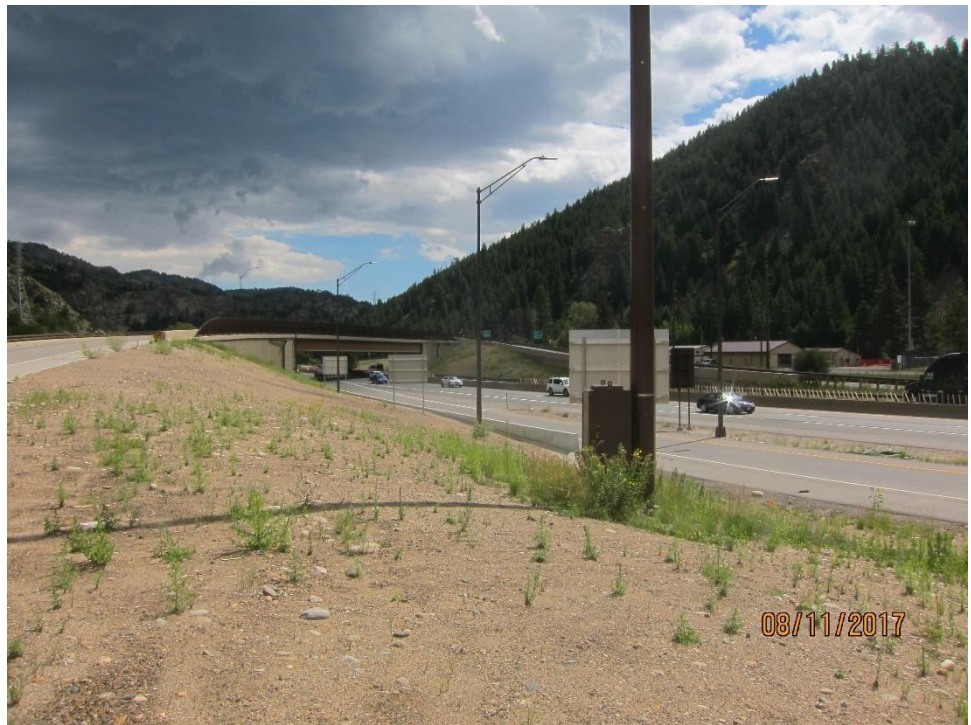
Overpass at I-70 exit 241.
