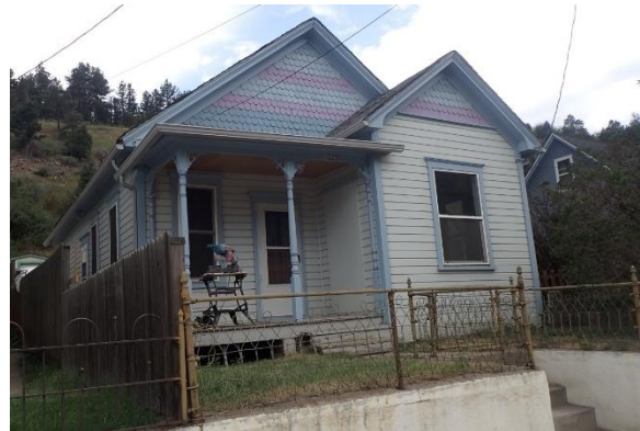
Photo 45. Façade (north) and east elevation of 2229 Miner Street.
