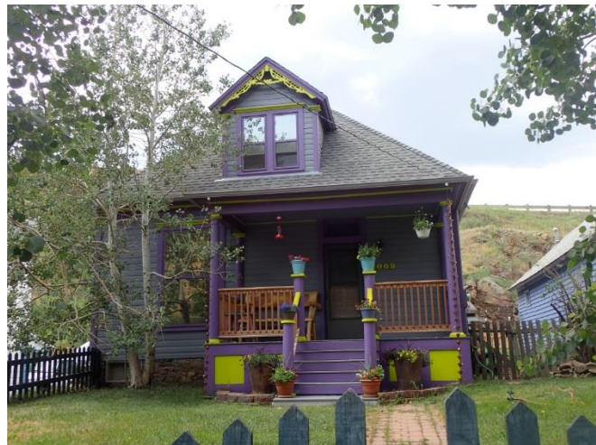
Photo 47. Façade (north) of 2009 Miner Street.
