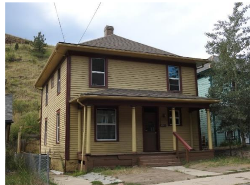
Photo 43. Façade (north) and East Elevation of the John Gunstrom House.
