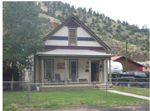
Photo 44. Façade (south) of 2730 Miner Street.
