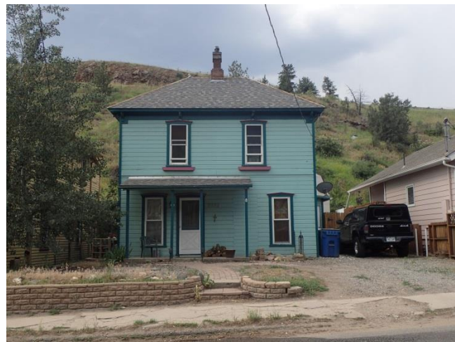
Photo 46. Façade (north) of 2023 Miner Street.
