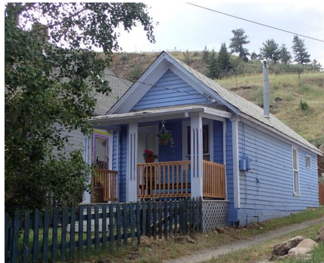
Photo 48. Façade (north) and west elevation of 2005 Miner Street.
