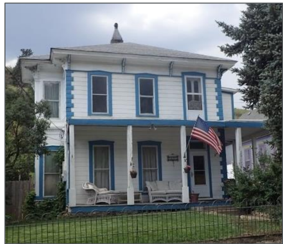
Photo 53. Façade of the Graham-Wilkins House (5CC.2475)
