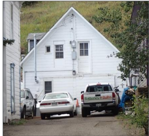
Photo 54. Primary (north) Façade of the Outbuilding (Garage) of the Residence at 2015 Miner Street (5CC.2475)
