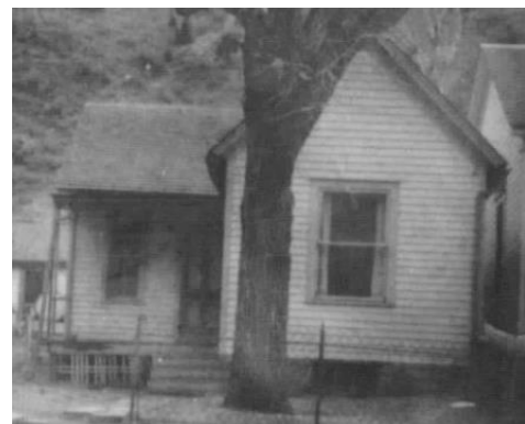
Photo 37. Original Construction of Residence at 2437 Miner Street (5CC.2453, circa 1950)
