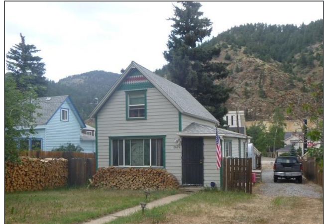
Photo 19. Primary (south) and East Elevations of the Residence at 2616 Miner Street (5CC.2439)
