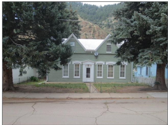
Photo 23. Primary (south) Façade of the Residence at 2608.5 Miner Street (5CC.2441)
