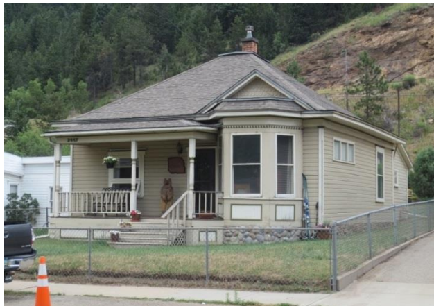
Photo 33. Primary (north) and West Elevations of the Residence at 2447 Miner Street (5CC.2451)
