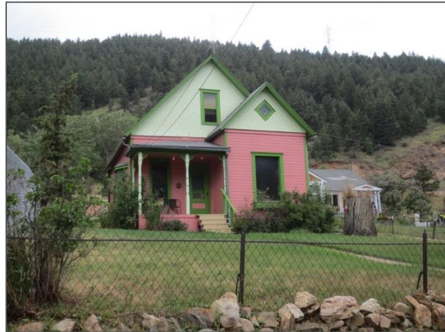
Photo 26. Primary (north) and East Elevations of the Residence at 2507 Miner Street (5CC.2445)
