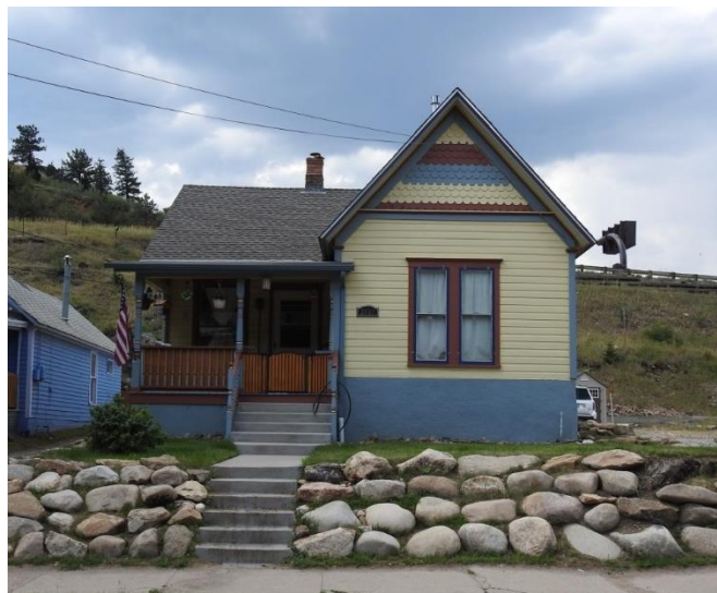
Photo 49. Façade (north) of 2001 Miner Street.
