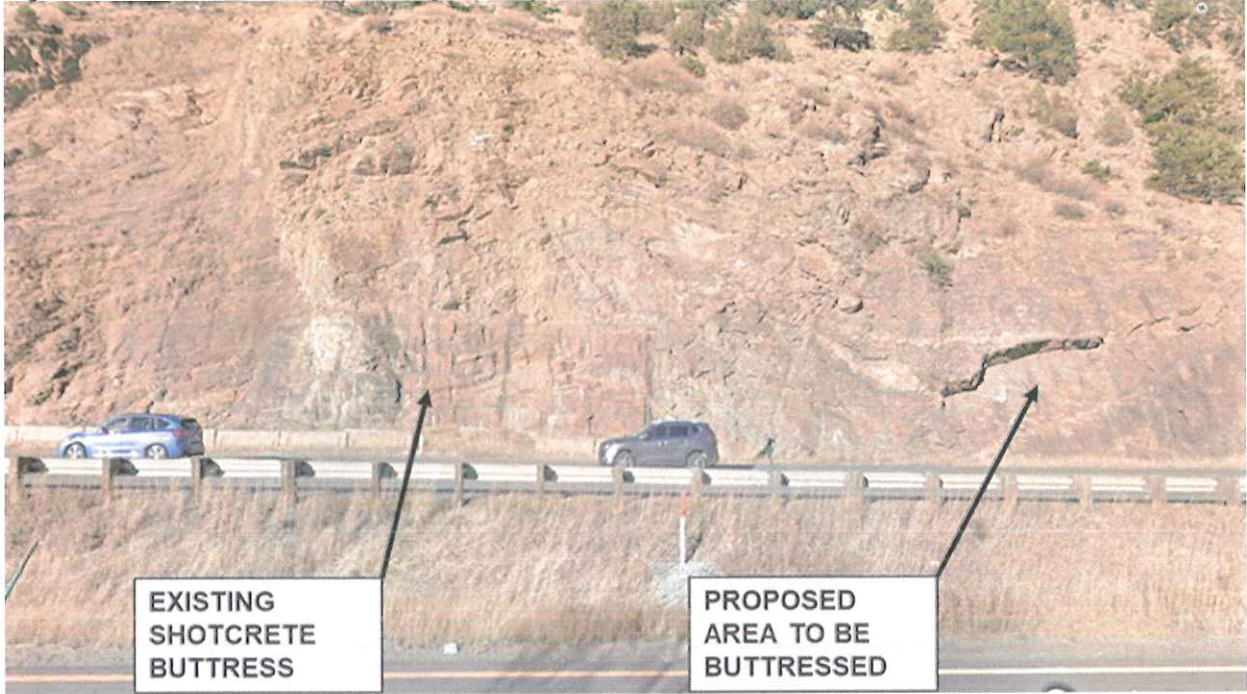
Figure 6. Location of Rock Buttressing Between Exits 238 and 239 with Adjacent Existing Buttressing.
