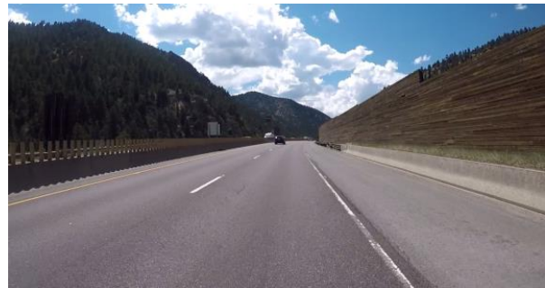
Photo 1. Existing Noise Wall at MP 239
