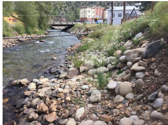
Photo 5. Looking north at Clear Creek in the town of Idaho Springs.
