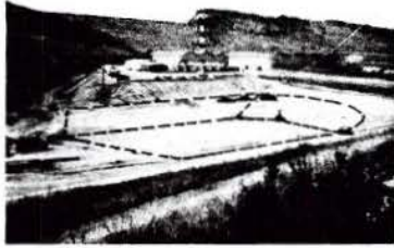
OVERALL VIEW OF FACILITY, AUGUST 1967
