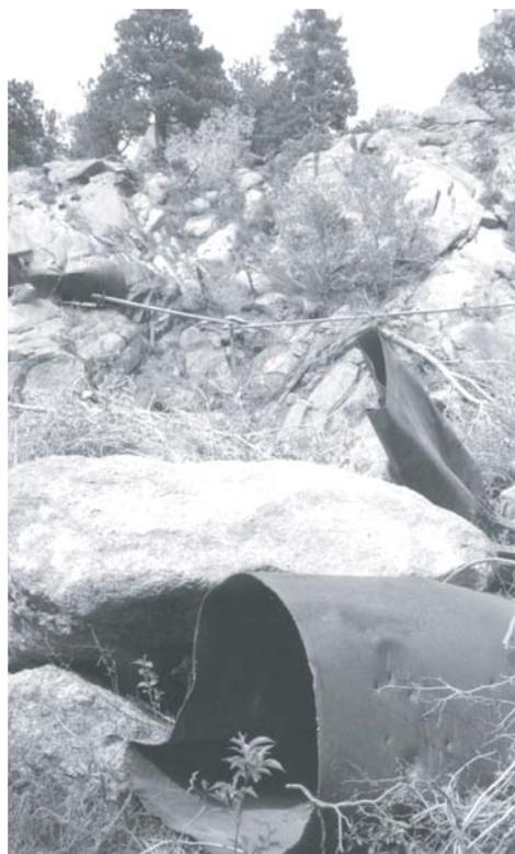
Destroyed flume from 1972, underneath the boulder culprit. Behind it is the pipe crushed in 1999.
