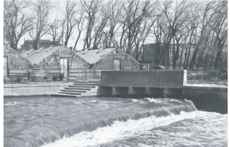
White Rock Ditch headgate and diversion dam, on whose design Frederick Law Olmsted, Jr. consulted. Photo 1921
