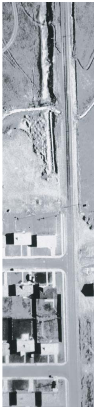
Anderson Extension Ditch (top) on its way into pipe (middle) under Martin Acres neighborhood (bottom), 1958
