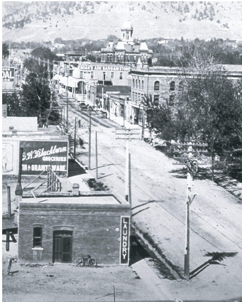
Laterals along Pearl Street, looking west from 17th Street, c. 1902
