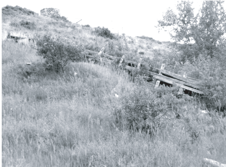
Ruins of the Farmers Ditch flume that crossed Six Mile Creek
