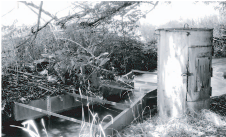
The Parshall flume and recording house for Silver Lake Ditch, 1999
