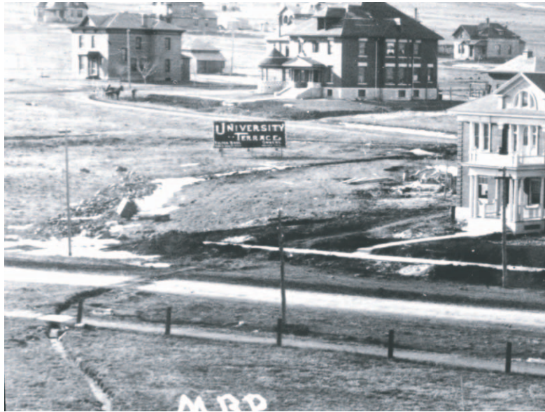
Lateral crossing Broadway to the campus, c. 1900. View from Hale Science (house at right is now parking lot at Pennsylvania Avenue).
