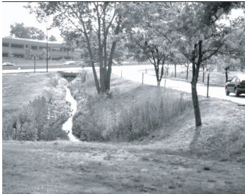
Anderson Extension Ditch daylights in the Table Mesa interchange.
