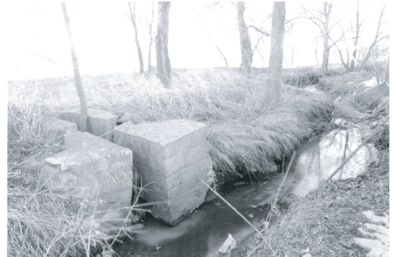
A remnant lateral headgate on the grounds of the new NOAA building, which irrigated what is now Martin Acres. Photo 1997.
