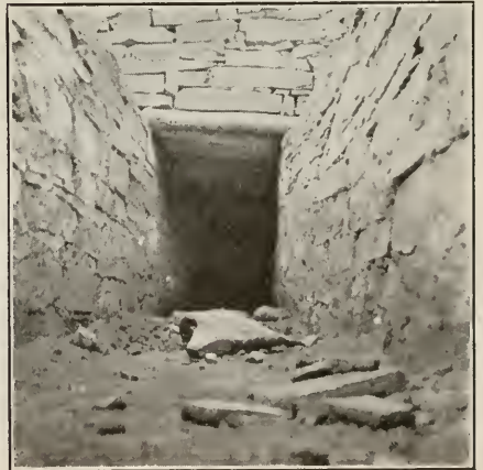
Upper Passage of the Double Ventilator
