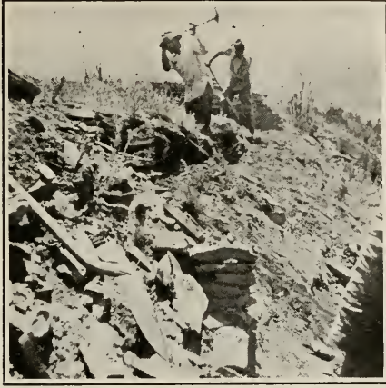
West End of Guardhouse Before Excavation
