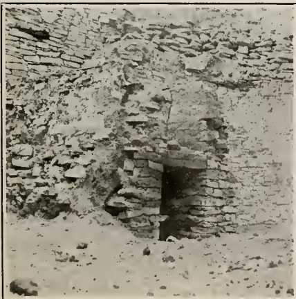
View of Ventilator From the Floor
