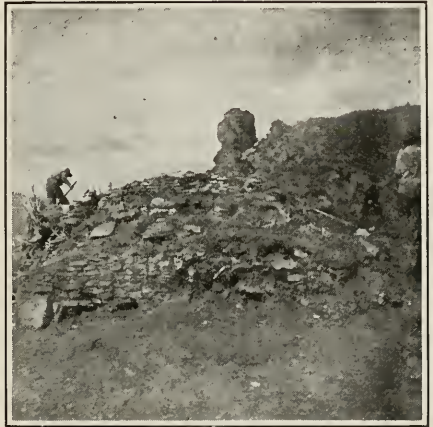
West End of Guardhouse After Excavation
