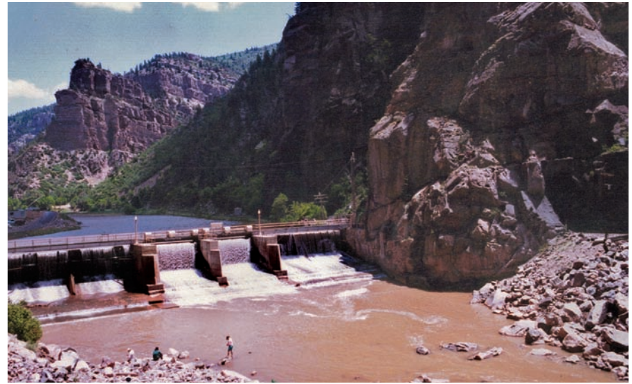
The Shoshone dam still diverts water into a tunnel for use at the downstream Shoshone generating station (15.0 MW capacity) using the drop in elevation in Glenwood Canyon as the power source. Photo Larry Scott.
