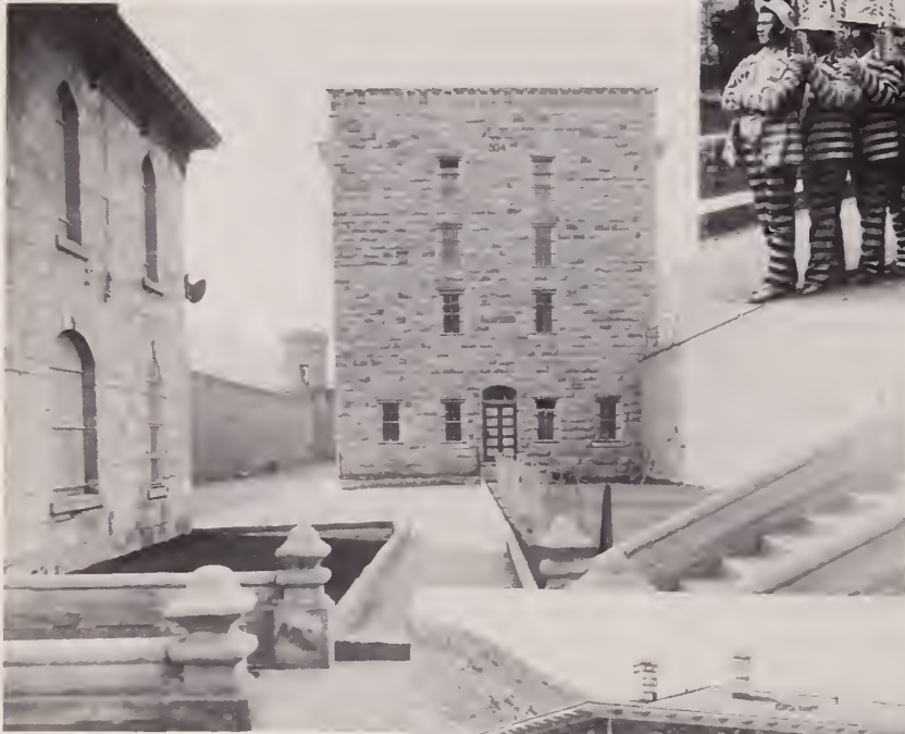
REAR OF ADMINISTRATION BUILDING and EAST END of CELLHOUSE #4
