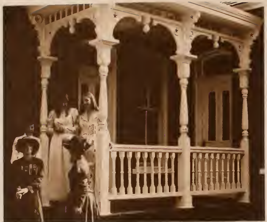
Centennial House After Restoration
