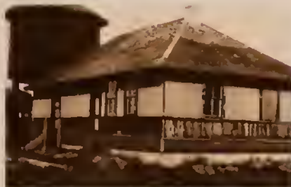
Gunnison Depot Before Restoration
