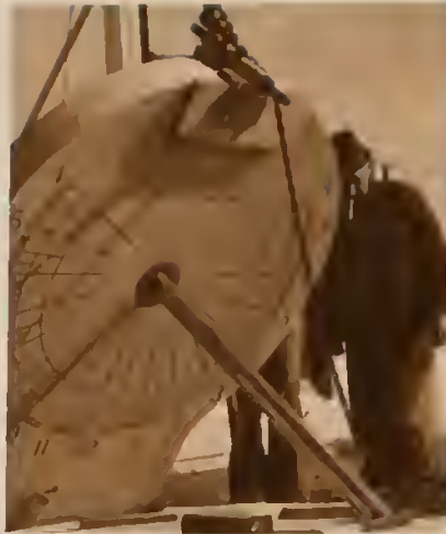
Installing the Sundial, Aurora
