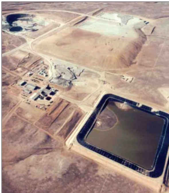
Figure 52. Aerial photo of a uranium mill. The mill itself, where the ore is crushed and the uranium and vanadium removed, is surrounded by a piles of the waste rock, from which the commodities have been removed, and a lined pond, containing water from the operation.
