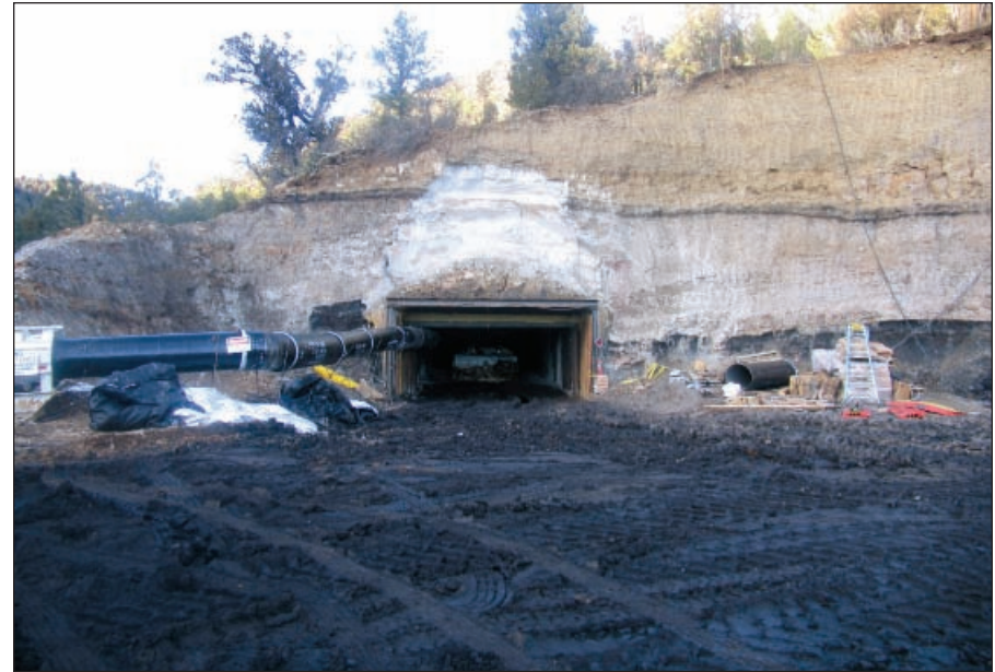
Figure 39. Construction activities at the new King II Mine, La Plata County. Shown are the main entry and ventilation systems. The coal bed is 6 to 7 ft thick, as shown in the cut slope face.
