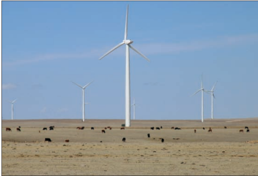
Figure 55. Cedar Creek Wind Energy Farm, Weld County. This wind farm has over 270 turbines generating 300 Mw capacity electricity when the wind is blowing, which is most of the time in northeastern Weld County.
