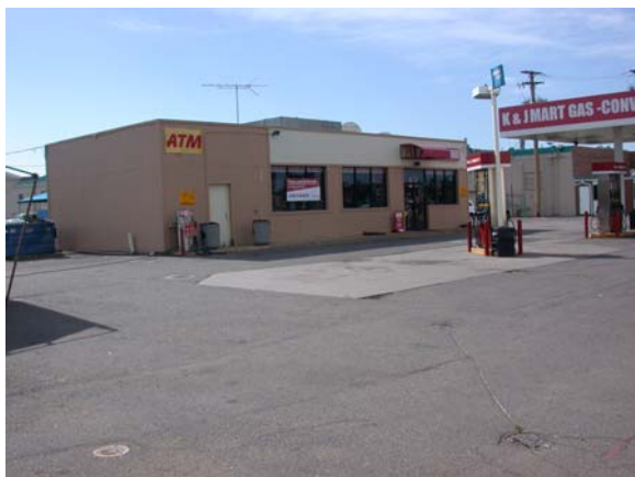
3. HH Texaco Service Station 5AH.3274 / 754 Peoria St. 1953
