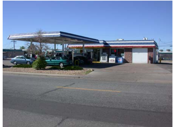
12. HH Phillips 66 Gas Station 5AH.3268 / 138 Del Mar Circle 1959
