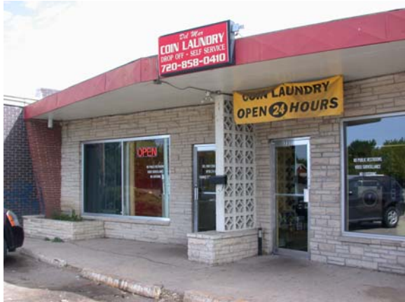
13. Swanson Retail Building 5AH.3264 / 122-124 Del Mar Cir. 1960
