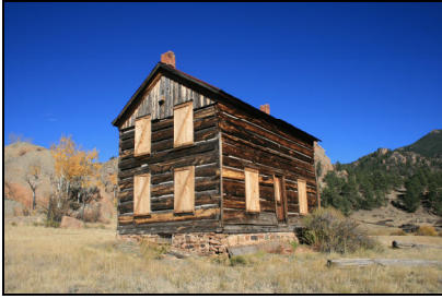
Williams Ranch, 25630 County Road 77, 5PA.38.
