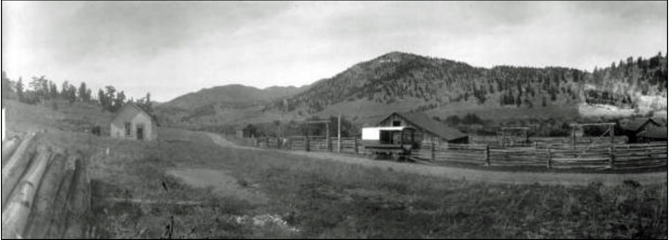
Figure 19. This view north along Tarryall Road from the Lazy River Ranch illustrates the landscape along the corridor in the early 1920s. The house on the left had not yet received its Rustic appearance. SOURCE: E.E. Van Epps photograph, image number 025-1833.jpg, Pikes Peak Library District, Colorado Springs, Colorado.
