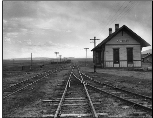
Figure 3. Railroads served the Tarryall Road corridor at its north and south ends. The Denver, South Park & Pacific Railroad built this frame depot at Jefferson, shown here at the time of the line's abandonment in 1937. SOURCE: Western History and Genealogy Department, Denver Public Library, M.C. Poor photograph, image number X-9576, June 1937.
