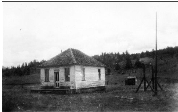
Figure 5. In this 1947 photograph Hayman school is shown in its second location, along Tarryall Road, after its days as an educational facility ended. Note the swingset to the right and a probable outhouse to the rear. SOURCE: Western History and Genealogy Department, Denver Public Library, Muriel Sibell Wolle photograph, image number X-5819, 1947.
