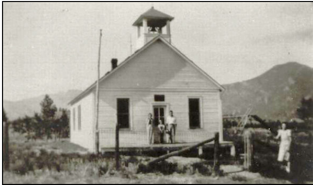
Figure 18. Listed in the National Register of Historic Places, the 1921 Tarryall School is representative of the one-room schools once found in rural areas throughout Colorado. SOURCE: Park County Local History Archives, image 300, provided by Sydney Johnson, 1941.
